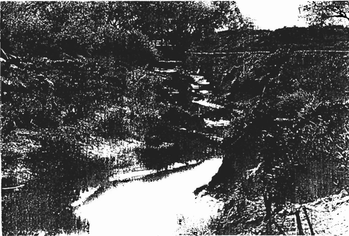
Same view, May 28, 1999. Note expanding point bar at Baffle 4, foreground. Point bar now at Baffle 3 in distance, and bank collapse in right foreground.
