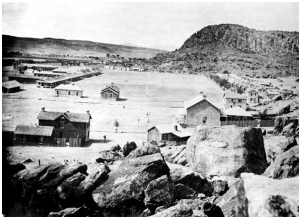
Figure 1. Historic Photograph Looking South with Chapel to the left of Flagstaff (c. 1886). Courtesy of Fort Davis NHS.
