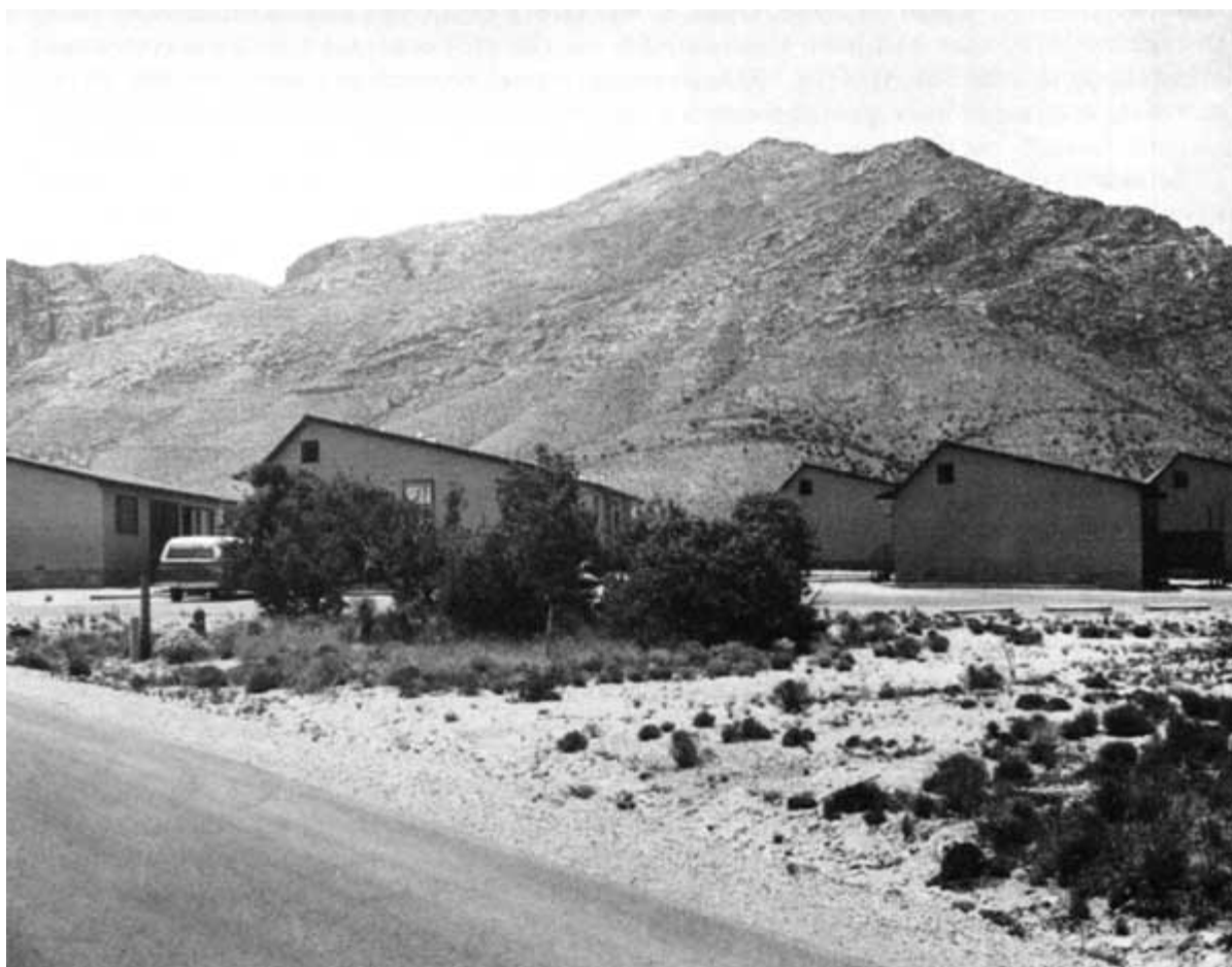
Figure 23. View of the duplex apartments, which are part of the permanent residential area built near Pine Springs, south of Highway 62/180. The residential area includes ten three-bedroom and two two-bedroom family units, two two-bedroom apartments, two studio apartments, and three duplex apartments. ( NPS Photo )
