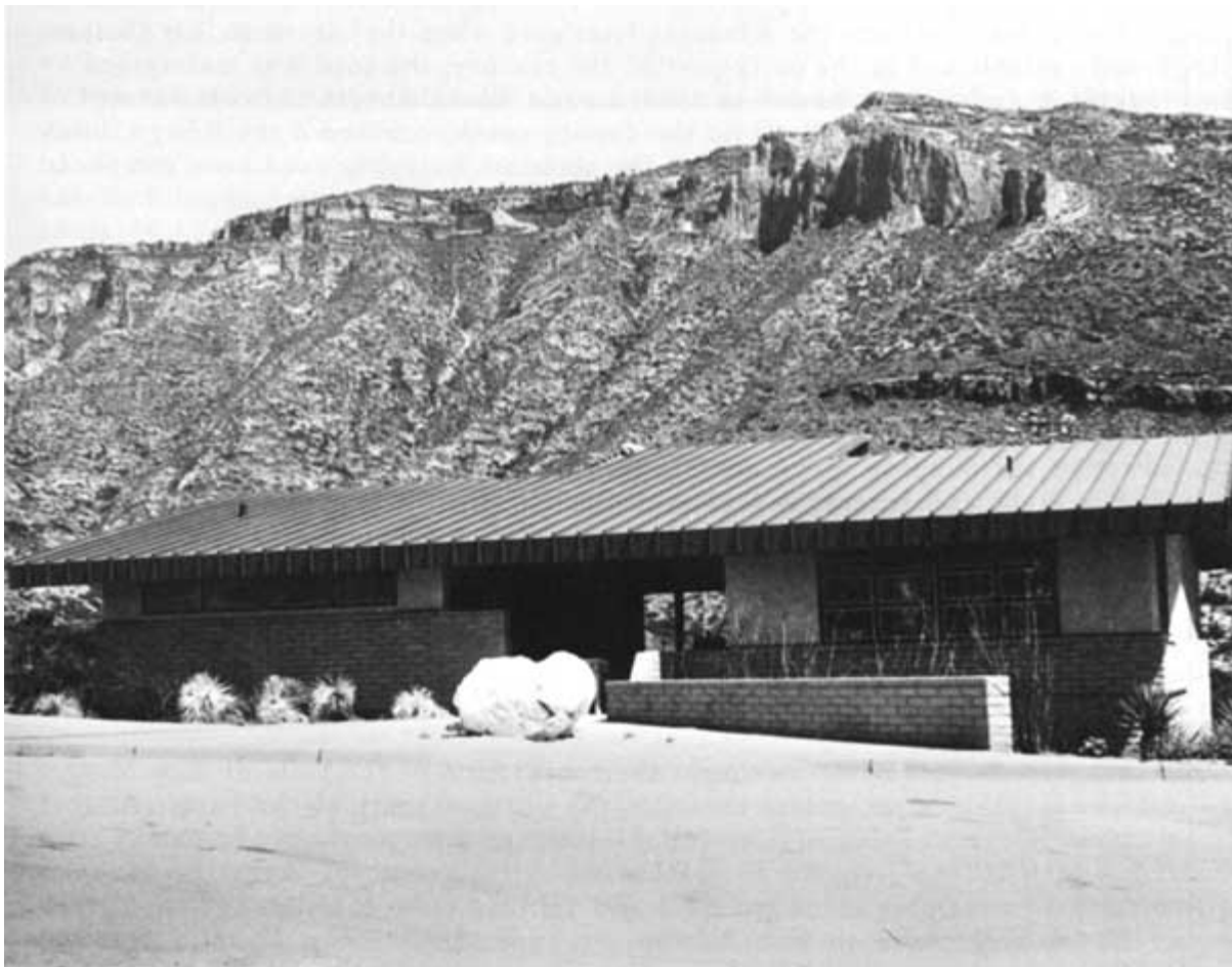
Figure 25. The permanent visitor contact station in McKittrick Canyon, completed late in 1982. Numerous problems plagued construction of this facility and delayed its completion by nearly two years. The contact station includes office and information space, restrooms, a patio area with exhibits, and an automatic audio-visual program with recorded narration by Wallace E. Pratt, donor of much of the land in McKittrick Canyon. (NPS Photo)
