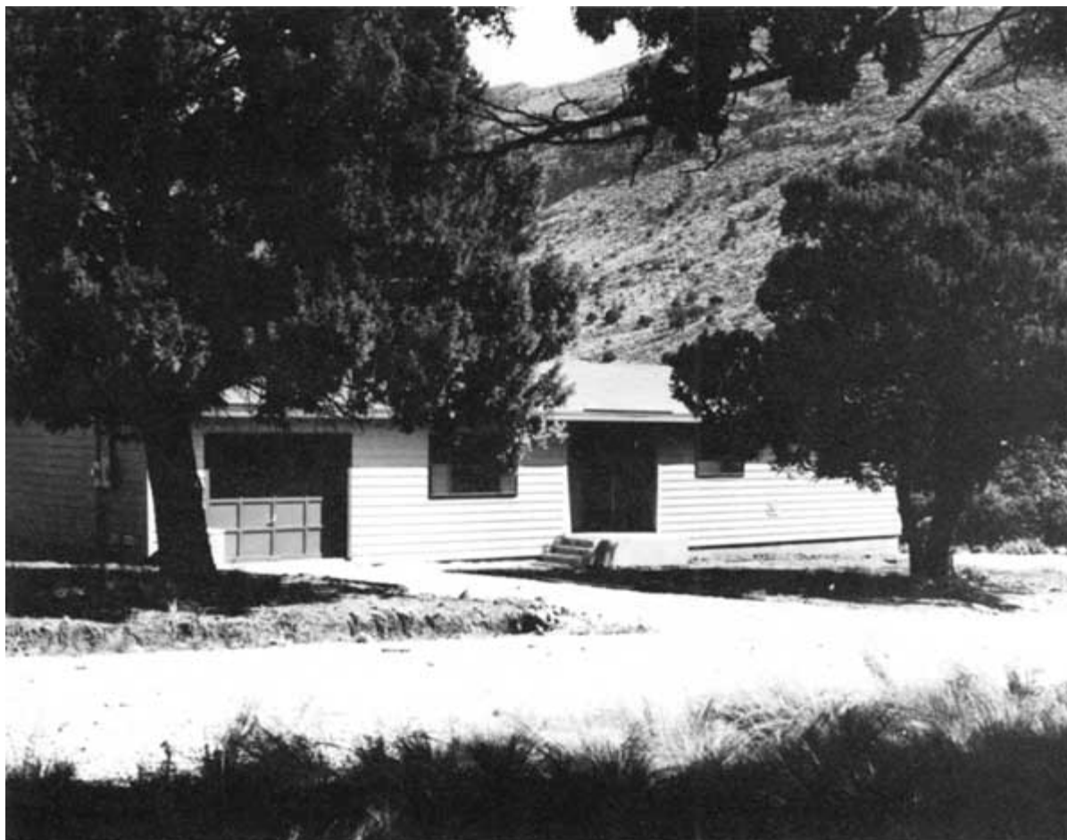
Figure 27. The new residence for the Dog Canyon ranger, completed in 1982. Planners located the house near the park entrance, on the west side of the road, a short distance from the campground area. (NPS Photo)
