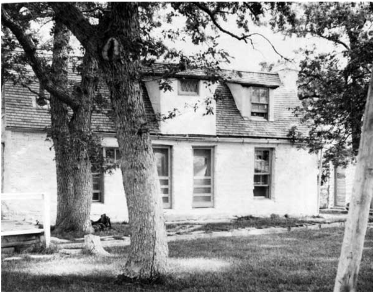
Figure 37. Frijole Ranch House, 1980. Listed in the National Register for its significance as a remnant of the early ranching economy in the Guadalupe, the Park Service has adapted the historic structure for administrative use. ( NPS Photo )
