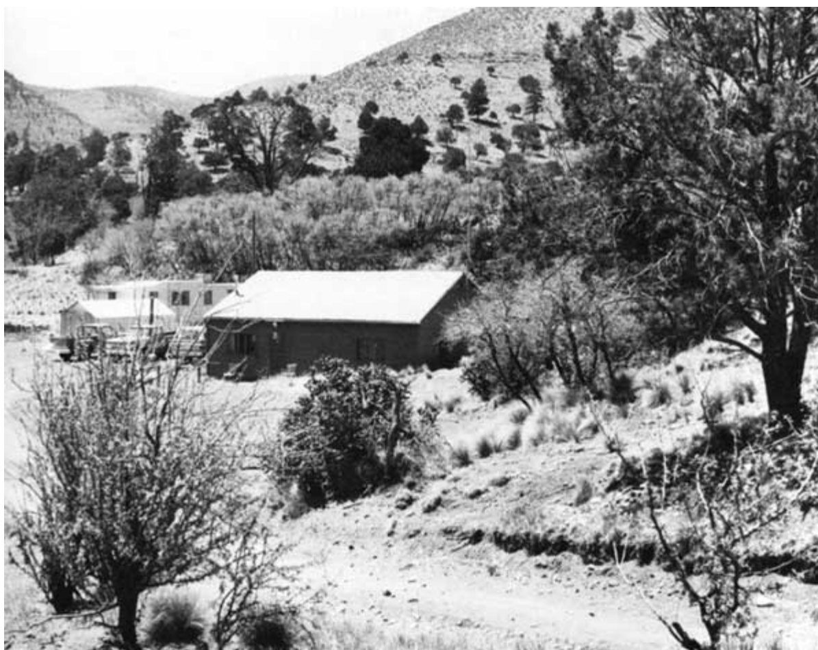
Figure 26. An existing ranch house and a trailer moved to the site by the Park Service served as ranger housing at Dog Canyon during the first decade of park operation. (NPS Photo)
