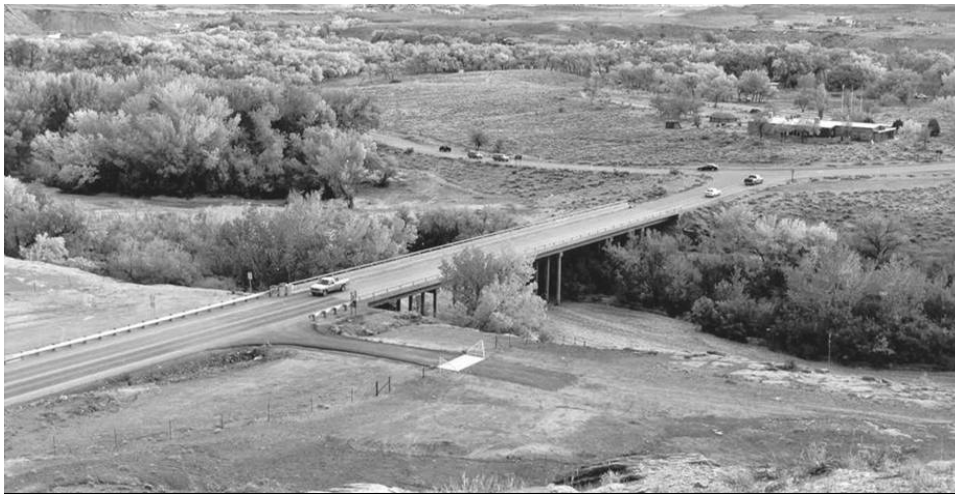
Figure 18a and 18b. National Park Service photo (top) and replicate photo (bottom) at the bridge over Chinle Wash.
