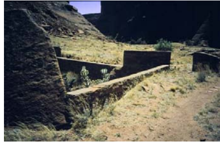
Figure 31, Small, old concrete dam near the mouth of Spring Canyon, Canyon de Chelly.
