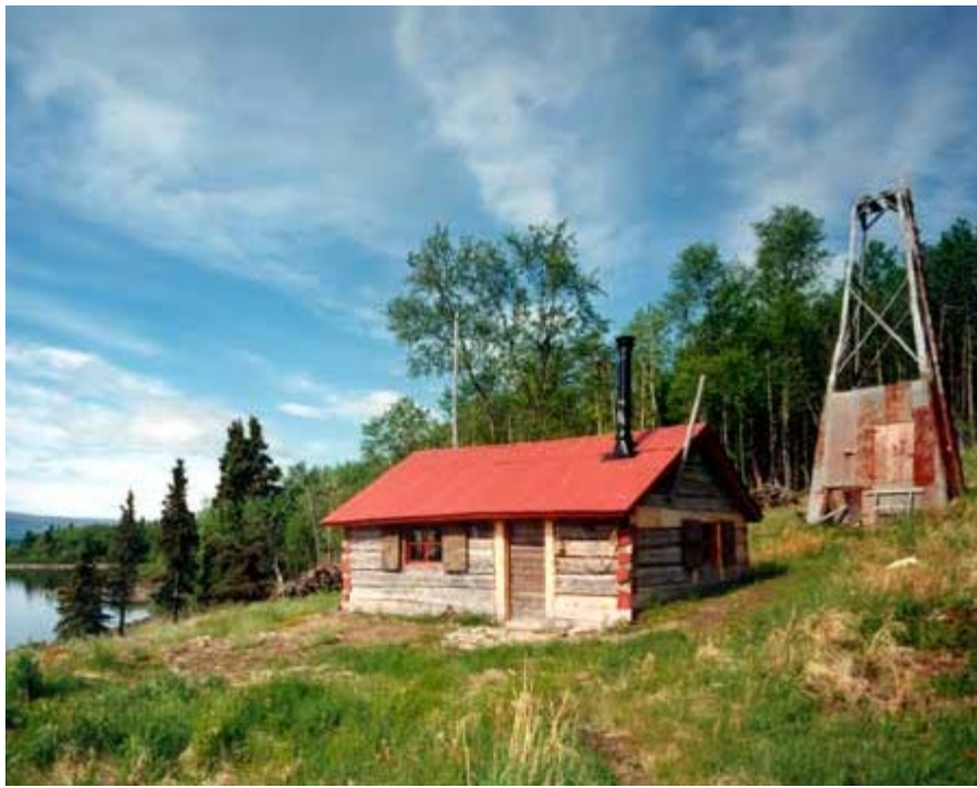
Roy Fures cabin at Bay of Islands. NPS-AKSO
