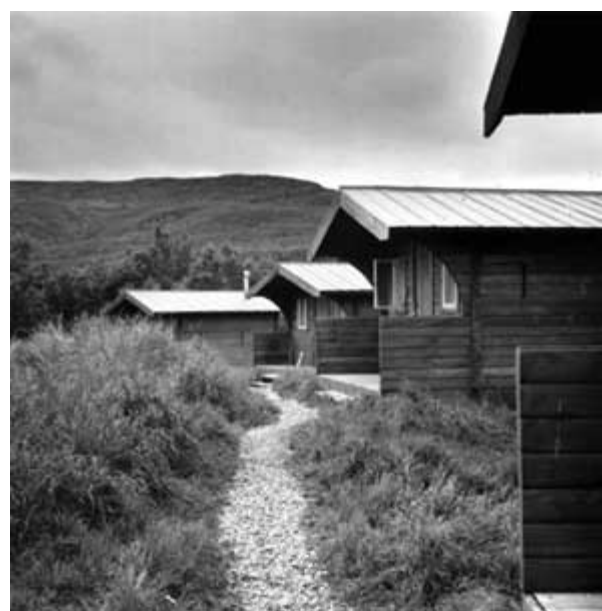
View of the Brooks Camp prefabricated Panabode guest cabins, built between 1960 and 1961. Looking northwest to Dumpling Mountain in 1971. Wien Collection, AMHA.
