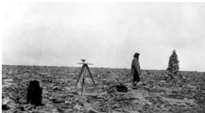
The National Geographic Society Katmai expedition members built rock cairns to use as survey reference points. This photo is titled "Station 24," which is believed to have been at or near the summit of Dumpling Mountain, 1918. Photo courtesy of University of Alaska Anchorage, Archives and Manuscripts Department, National Geographic Society Katmai Expeditions Collection, Box 4, 3614.
