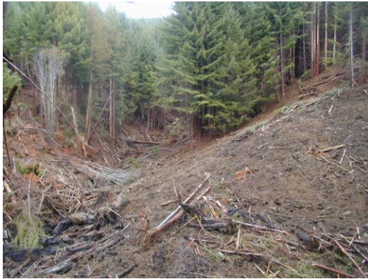
Photo 5: Post-excavation view of RX3, looking upstream. Photo taken from a mid-point between the two excavations of RX3 and RX4. Prominent fillsite for this and RX4 excavations is located along the right portion of the photo.
