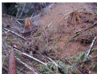
Photo 12: Post-excavation view of RX E1, taken from lower right side of excavation looking upstream.
