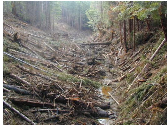
Photo 8: Post-excavation view of RX3, looking from top towards the bottom of the excavation. Pooling water are sections where large woody debris was used to arrest material left in the channel.
