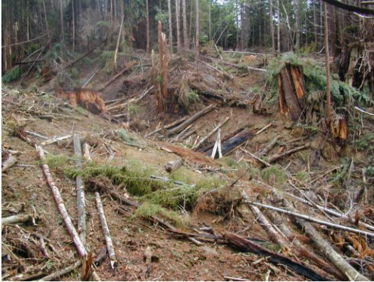
Photo 2: Post-excitation view of RX1 from right side of excavation. Fillsite for both RX1 and RX2 located to the left of the photo, above the confluence of the two stream crossings.
