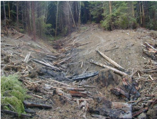
Photo 16: Post-excitation, early winter view of RX W2, taken from the lower right bank of excavation looking upstream.
