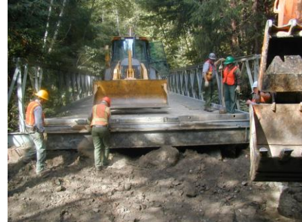
Photos show the Bailey bridge, at right, and the work crew beginning to prepare for removal and disassembling the bridge.
