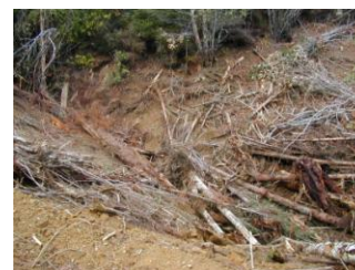
Photo 13: Post-excavation view of RX E2, taken from lower right side of excavation looking upstream.
