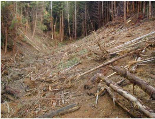
Photo 7: Post-excavation view of RX3, looking from bottom of excavation towards the top.
