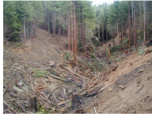
Photo 6: Post-excavation view of RX4, looking upstream. Exposed slope along right side of photo is referenced in narrative on excavation and is the location where post-excavation adjustment was most pronounced.
