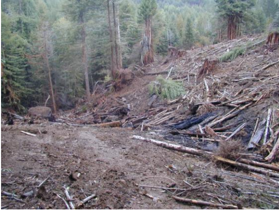
Photo 14: Post-excitation, early winter view of RX W2, taken from the upper right bank of excavation looking downstream.
