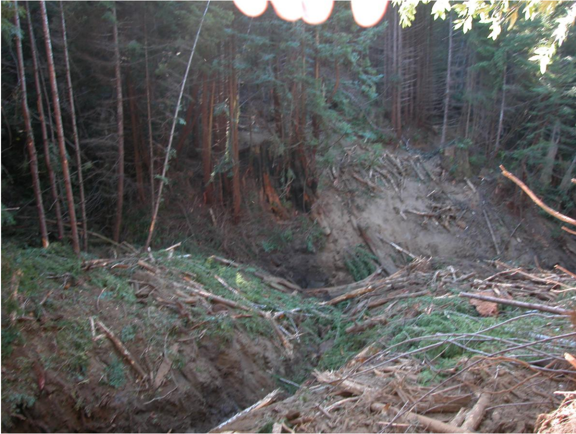
Figure 11. Looking down stream at the west bank (left bank of Upper Y) where a portion of the B551b was removed during the Upper Y excavation. Additional brush mulch was applied during the removal of the remaining B551b, covering the bare slope seen in this photograph. Photo location PP0303031b.
