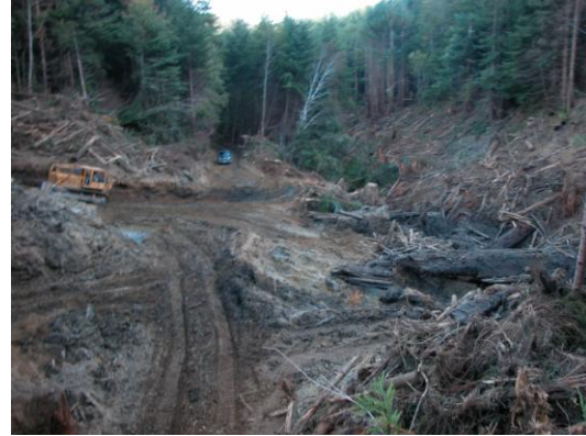
Figure 17b. B540 Landing with main channel excavated.
