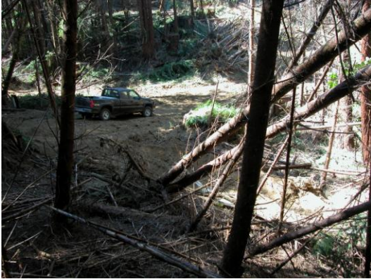
Figure 12a, Photo point 030305-1 as the lower Y crossing (Work Item 5) was being cleared prior to excavation.
