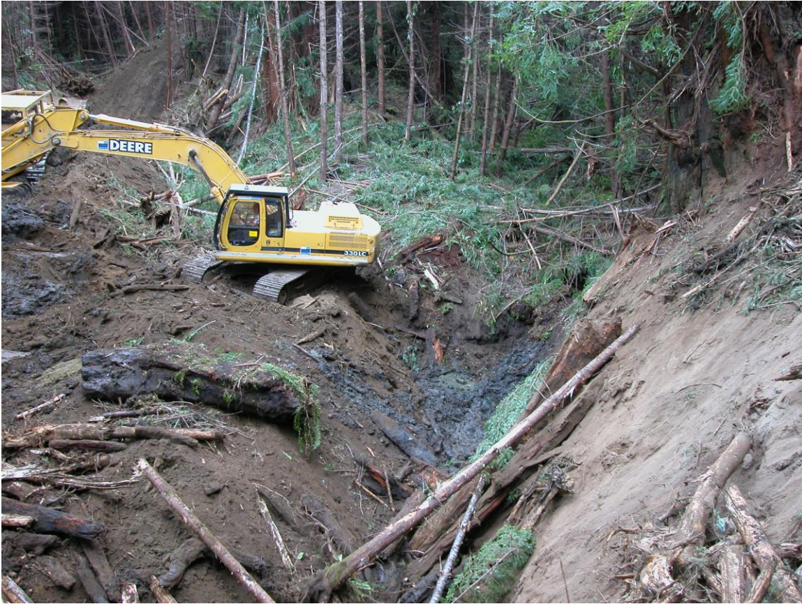
Figure 10, Looking upstream at the confluence of east and south forks at Upper Y crossing. Minimal fill in the south fork (to the right of the excavator) reduced the cost benefit ratio resulting in leaving the fill to adjust through runoff processes.
