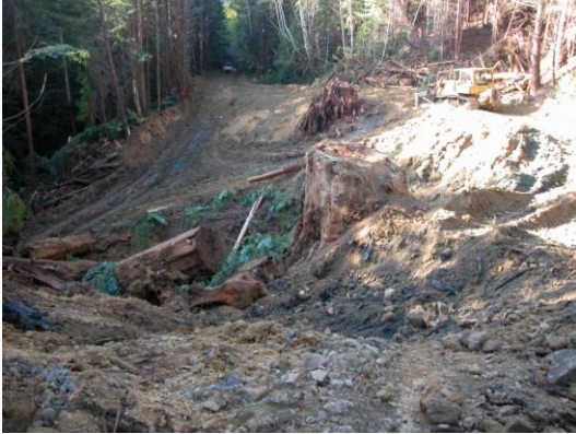
Figure 19a. Hollywood Bowl, partially excavated, dozer on B500 road elevation.
