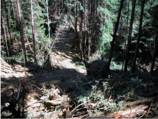
Figure 15a. Push road that was rebuilt to transport fill across mainstem, through RX4.
