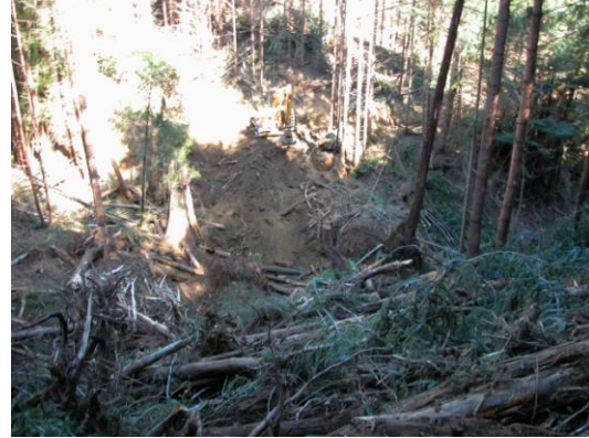
Figure 15b. Excavation of last portion of fill from mainstem channel at RX4.
