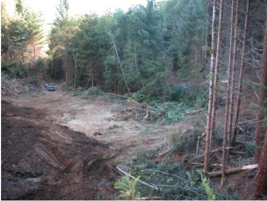
Figure 17a. B540 Landing during early excavation.
