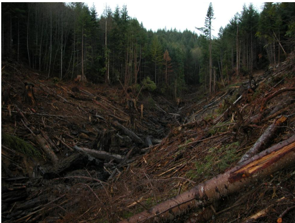
Figure 11. RX16 (Work item 16) finished slopes viewed from the lower left bank looking upstream to the top of excavation. The enormous in-place stump is in the left center of the photo.
