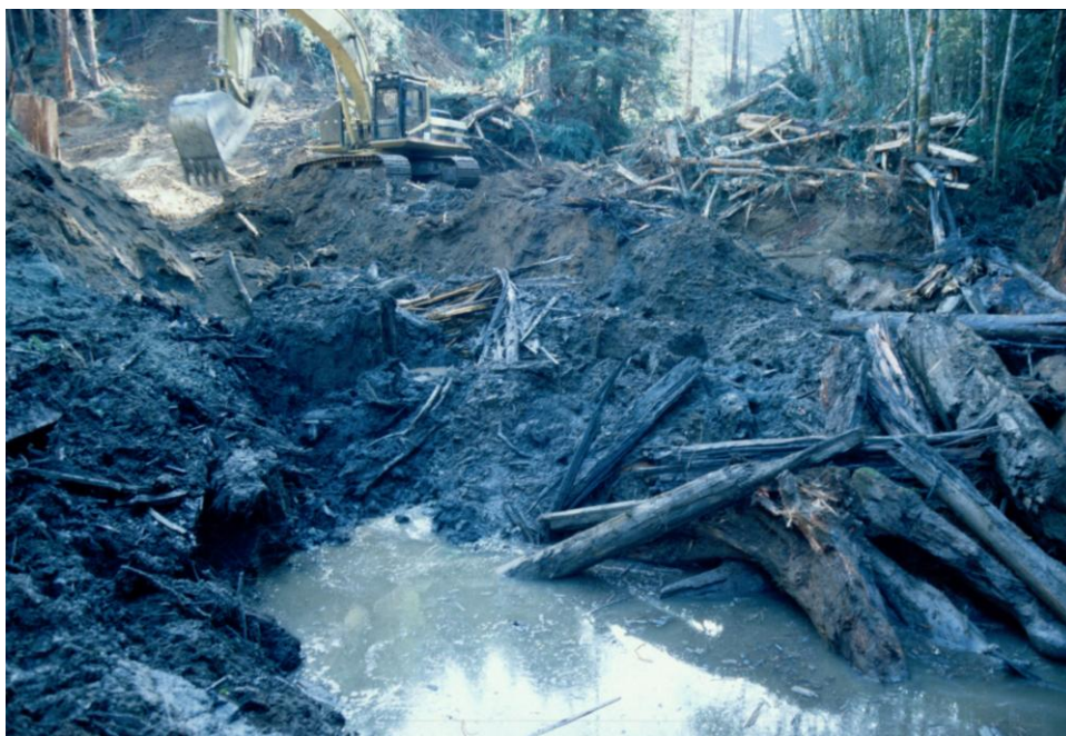
Figure 8. RX3, Work Item 7, during excavation viewed from the lower left bank. The bluish unconsolidated gravel can be seen above water level and
