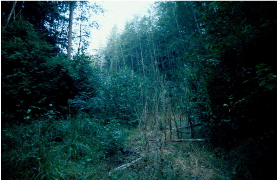
Figure 4. Pre-excavation view of RX1, Work Item 3, looking downstream from the middle of the Larry Damm Creek debris deposit just upstream its the confluence with Rx-1's creek. The right side of the image is a 20 foot high wall of fill covered in vegetation.
