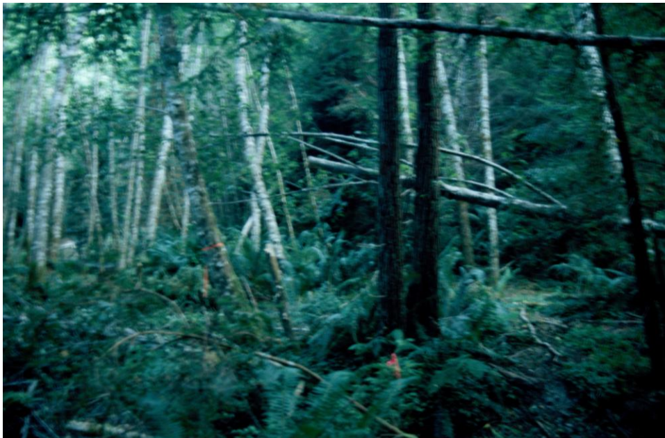
Figure 6. RX3, Work Item 7, prior to excavation viewed from across Larry Damm Creek. The view is up towards the confluence of the two tributaries.
