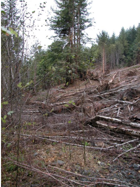
Figure 5. The finished slope of RX1, Work Item 3, looking downstream from the middle of the Larry Damm Creek debris deposit just upstream its the confluence with RX-1's creek. The wall of fill has been removed and the finished surface covered with vegetation.
