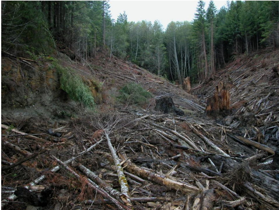
Figure 9. RX3, Work Item 7, finished slopes viewed from the lower left bank up to the top of RX3. The springy cutbank is on the center left edge of the photo and the settling pond is just out of view in the bottom right corner.
