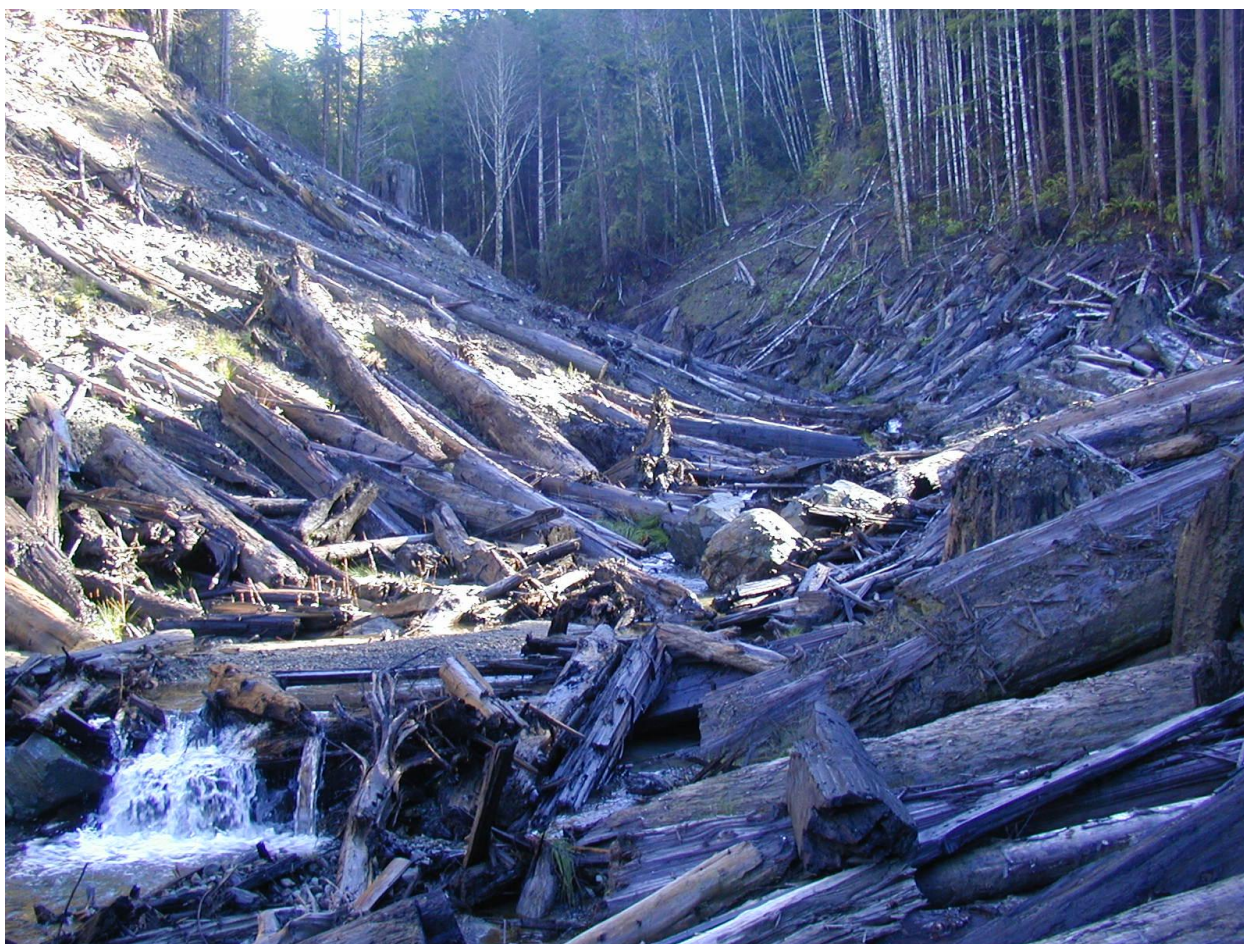
Figure 4. A stream crossing excavation with extensive woody debris placement. This photo was taken after the first winter following excavation. Adaptive Management
