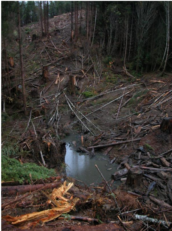
Figure 10. Fillsite to southwest of RX16. Finished slopes viewed from the lower left bank looking downstream. Settling pond is in the lower center and the unexcavated right fork is in the middle right of the photo.
