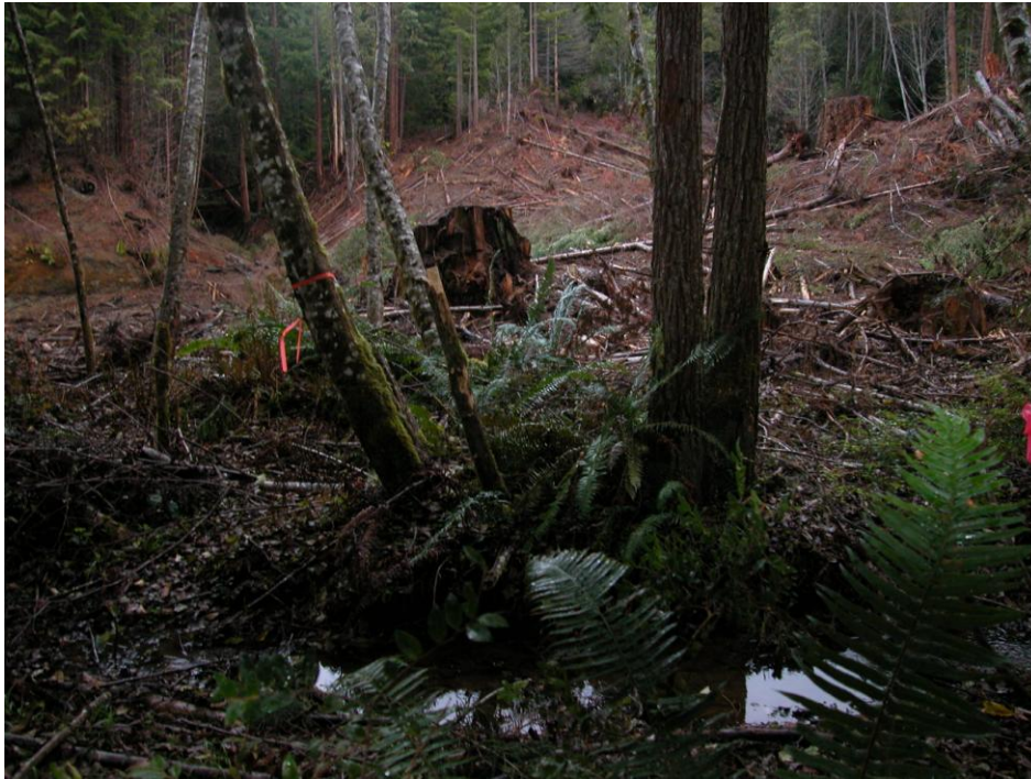
Figure 7. RX3, Work Item 7, after excavation viewed from across Larry Damm Creek. The view is up towards the confluence of the two tributaries. Notice the twin second growth redwoods in Figures 6 and 7.
