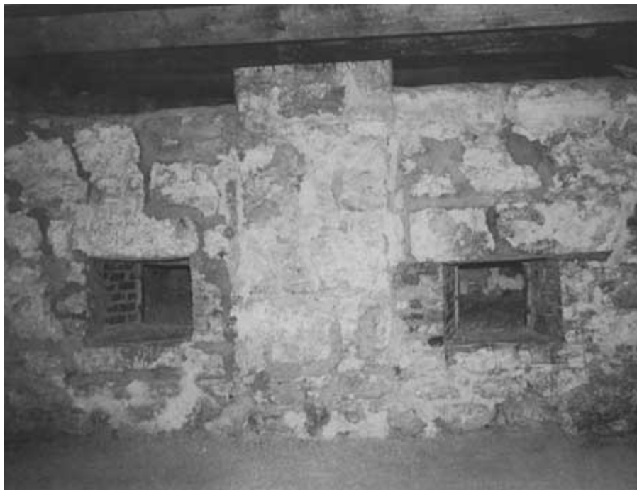
Plate III. Reconstructed H.B.C. bake ovens in Northwest Bastion, Lower Fort Garry, originally built c. 1846-1848. The doors to these ovens are only 24 inches above the floor. One chimney serves both ovens. ( National Park Service photograph by A. L. Koue, September, 1967. )
