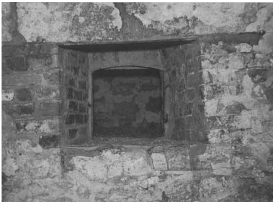
Plate IV. Oven entrance details, Northwest Bastion, Lower Fort Garry. The vaulted ceiling of the baking chamber is 3'3" high at the top of the arch. ( National Park Service photograph by A. L. Koue, September, 1967. )
