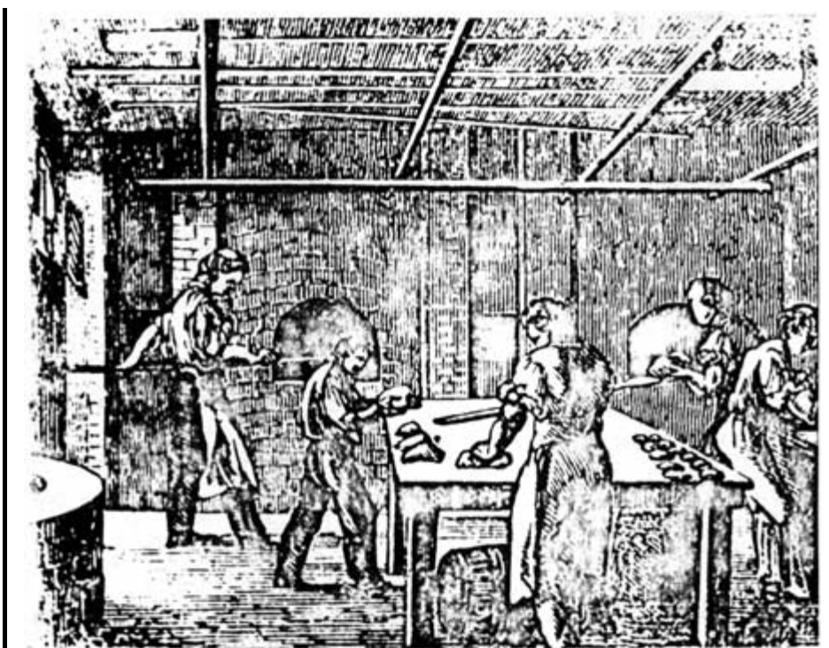
Figure 11. A two-oven bakehouse in 1842. The circular stone or brick structure on the left evidently is the fireplace for heating the "copper" or "cauldron." Note the position of the table between the two ovens and the ceiling racks for the peels. (From Panschar, Baking in America , I, facing p. 32.)
