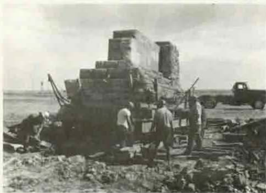
Illus 4. Pylon being moved from east entrance to Painted Canyon overlook (photograph from park files, taken August 1968)
