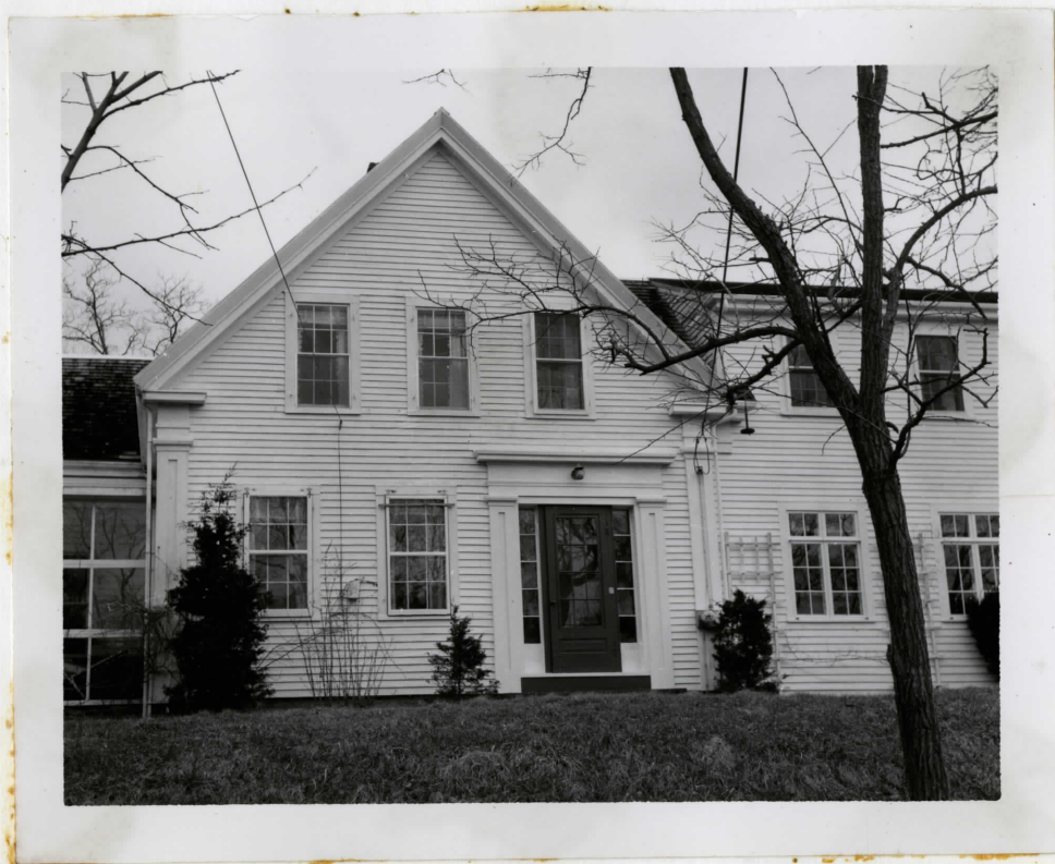
Old Center Section (c. 1850) with portion of West Wing (left) and East Wing (right)
