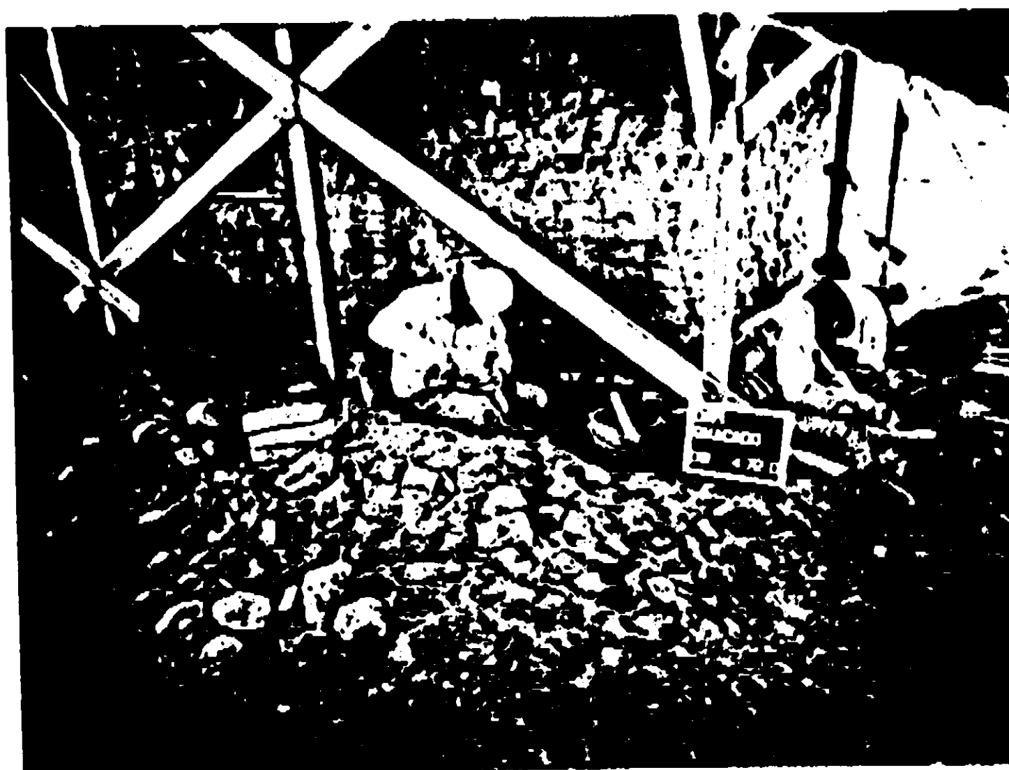
The original margins of the masonry is easily seen in the top photograph (see arrow.) In the lower photo workers are repairing a badly undercut corner.
