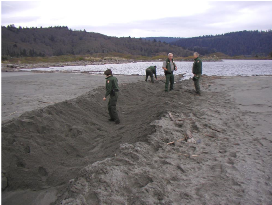
Figure 10. Filling in the illegally dug channel to stop the water flow (October 27, 2005 RNSP).
