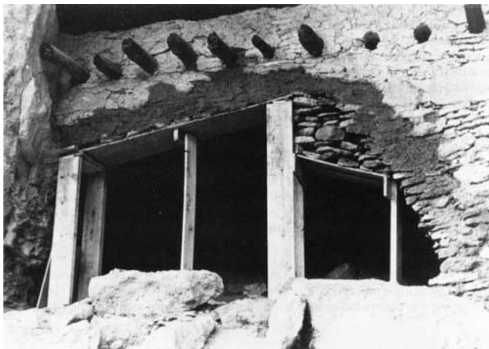
The archway in Cave 3 was stabilized with a metal rod and cement in 1963. Visitors enter the ruin through this arch. In 1968, the addition of a ladder descending from Cave 4 permitted a one-way path for people to walk through the ruins. Note the threatening cavity beneath the two-story structure.
