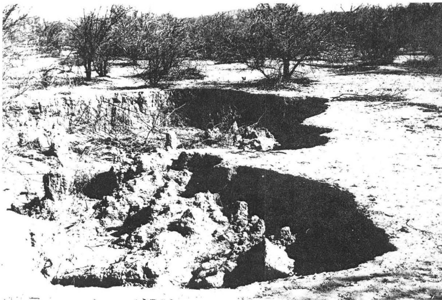
Fig. 45. Head of channel cutting 150 meters south of the Armenta Well enclosure. The channels are approximately 0.9-1.2 m deep. Photographed 1 December 1975
