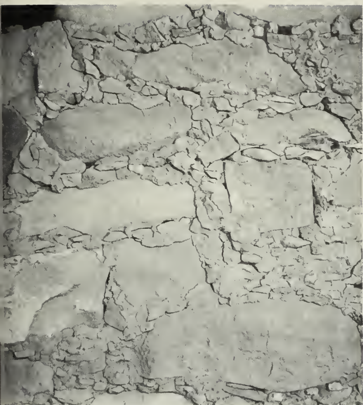
Figure 19—Scabbled masonry wall: stones are shaped but pecked or ground on the surface. Site 1202.
