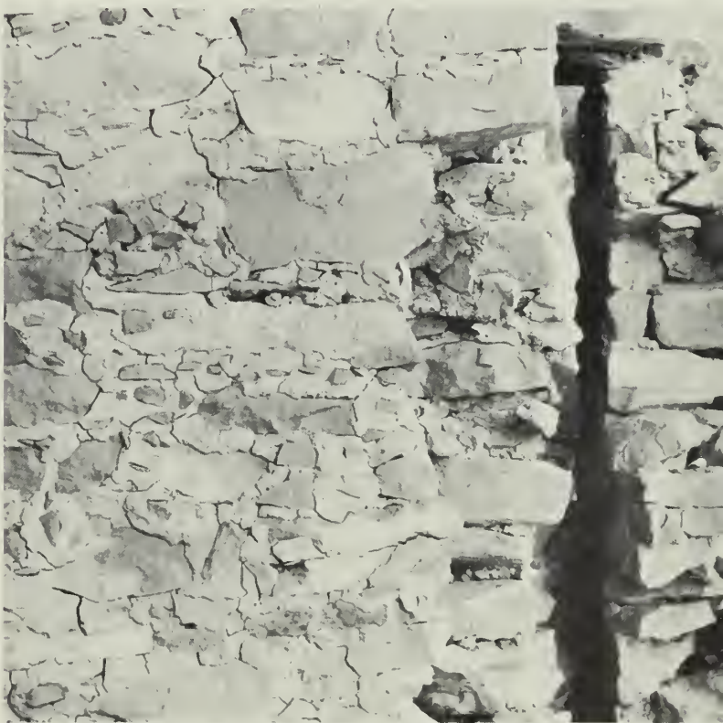
Figure 25—Exposed section of compound wall. Site 1355.
