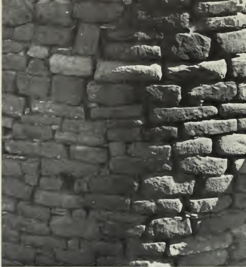
Figure 20—Finished masonry. Pecked surfaces of rock in classic wall of tower on Wildhorse Mesa. Site 1138.
