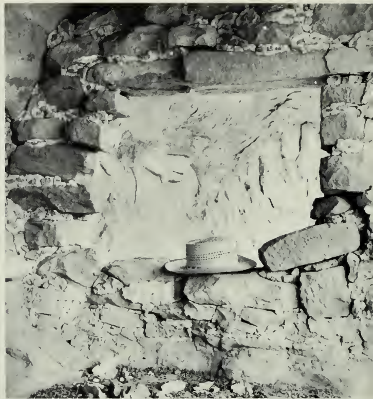
Figure 18—Scabbled stone wall in small cliff dwelling in Bobcat Canyon. Site 1373.
