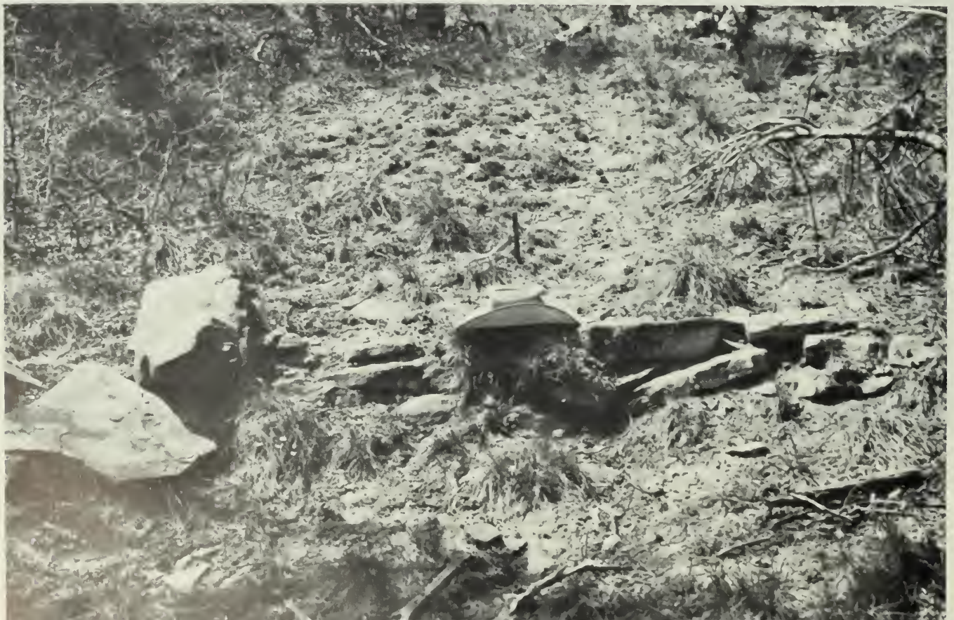
Figure 72—One of a series of 25 check dams. Site 1539.
