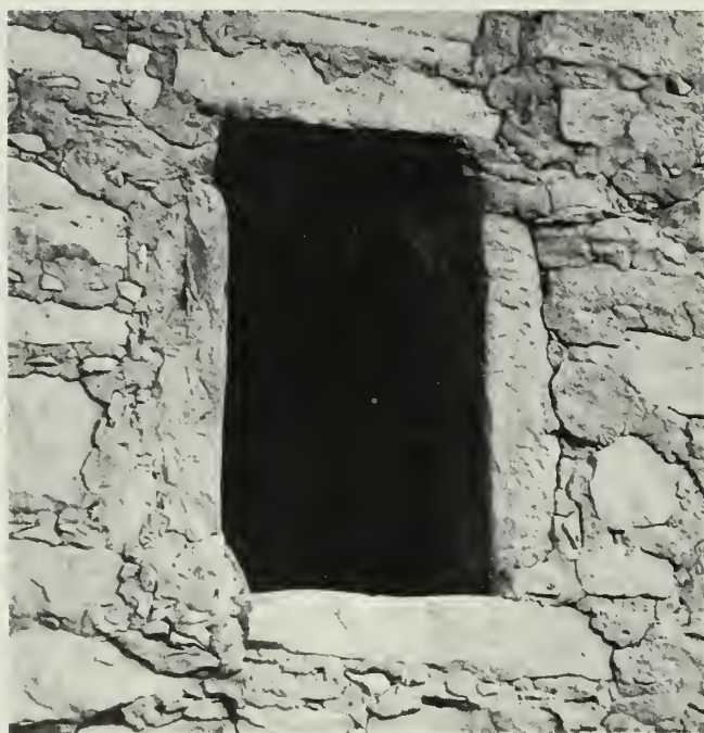
Figure 115—Doorway with digging stick used as false lintel or stop for slab door. Site 1221.
