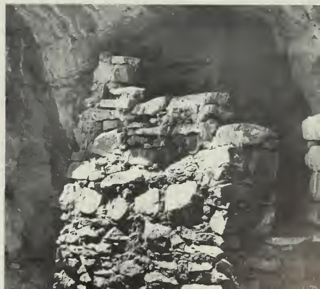
Figure 16—Rough wall, 2 or 3 stones showing some scabbling. Site 1266.
