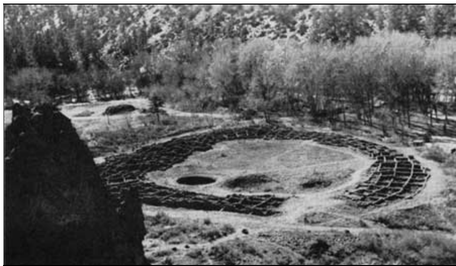
FIG. 38. TYUONYI AFTER STABILIZATION.
