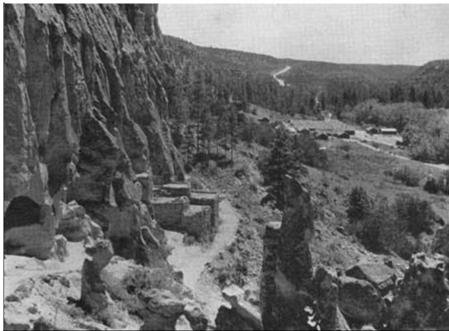
FIG. 41. VIEW OF NORTH CLIFF SHOWING RECONSTRUCTION OF TALUS HOUSE.
