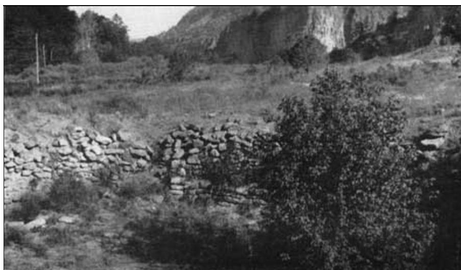
FIG. 6. LARGE KIVA BEFORE STABILIZATION. NOTICE UNEXCAVATED WEST ENTRANCE IN WALL.
