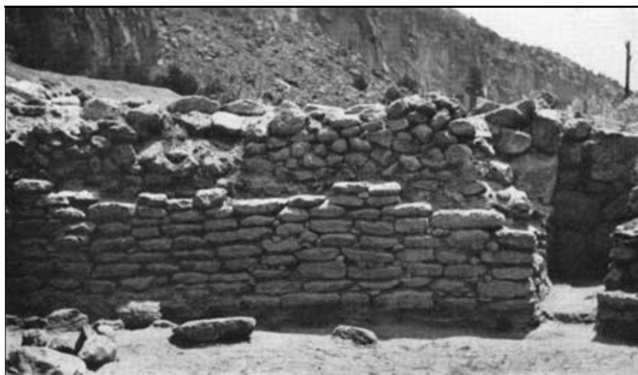
FIG. 7. VENTILATOR SHAFT AFTER CLEANING AND A SECTION OF DOUBLE WALL.
