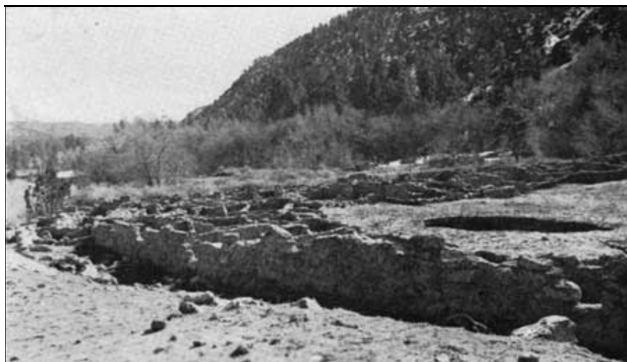
FIG. 36. NORTH AND EAST SECTIONS OF ROOMS AFTER STABILIZATION.
