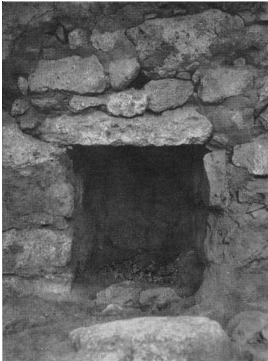
FIG. 26. STABILIZED VENTILATOR SHAFT OPENING IN CEREMONIAL CAVE KIVA.
