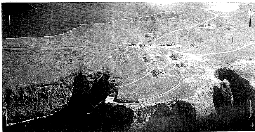
Fig. 20. Close-up of the Lighthouse Service installations that appear to have been augmented by the Navy. This is on the easternmost island of the Anacapa group. Location of military and Lighthouse Service facilities at this end is fortunate in that it insures that the main portion of the island will remain comparatively free from disturbance. Whether the flat, light-colored area at the upper right is a water catchment basin or a landing strip for small liaison planes was not learned.
