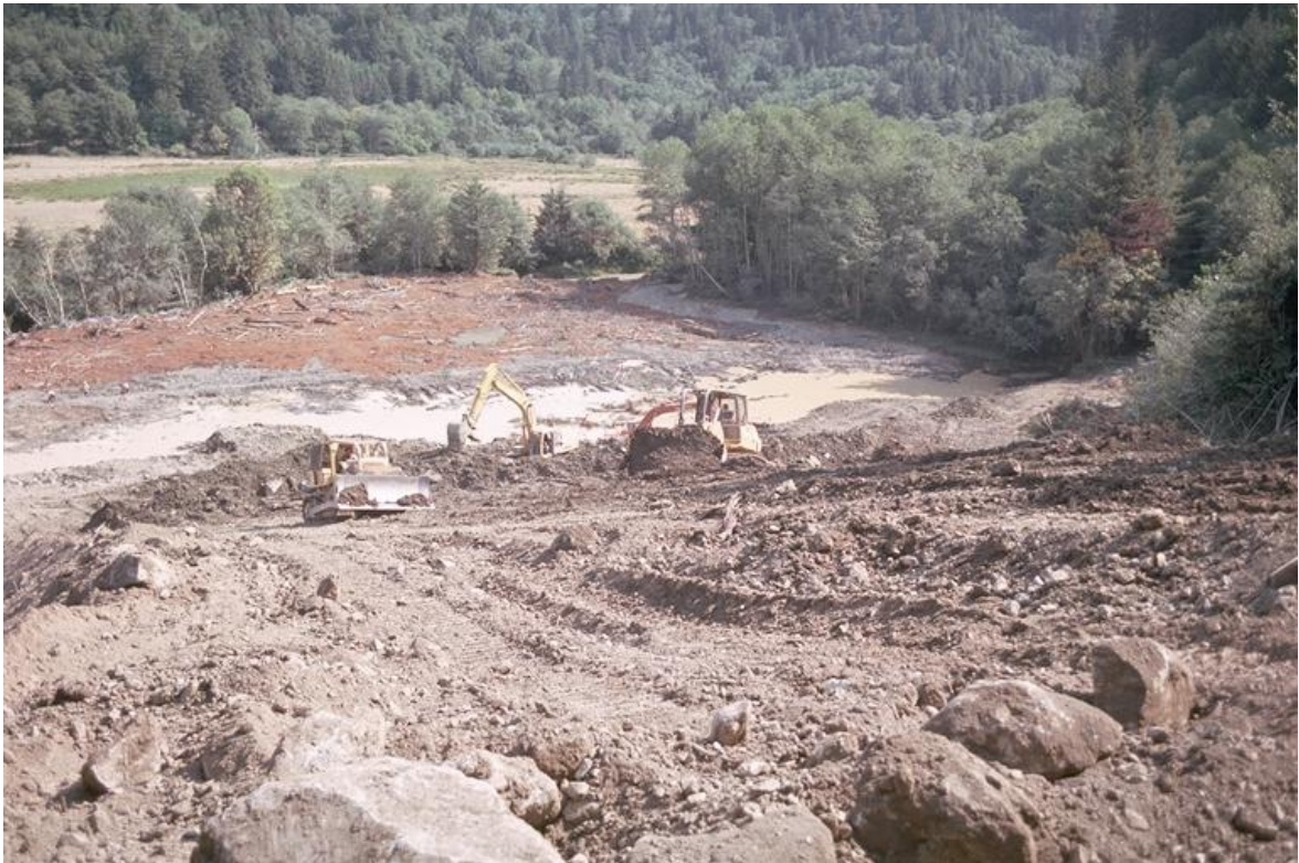
Photo 2. Rocks in foreground (averaged 18 to 48 inches in diameter), frequently encountered during excavation.
