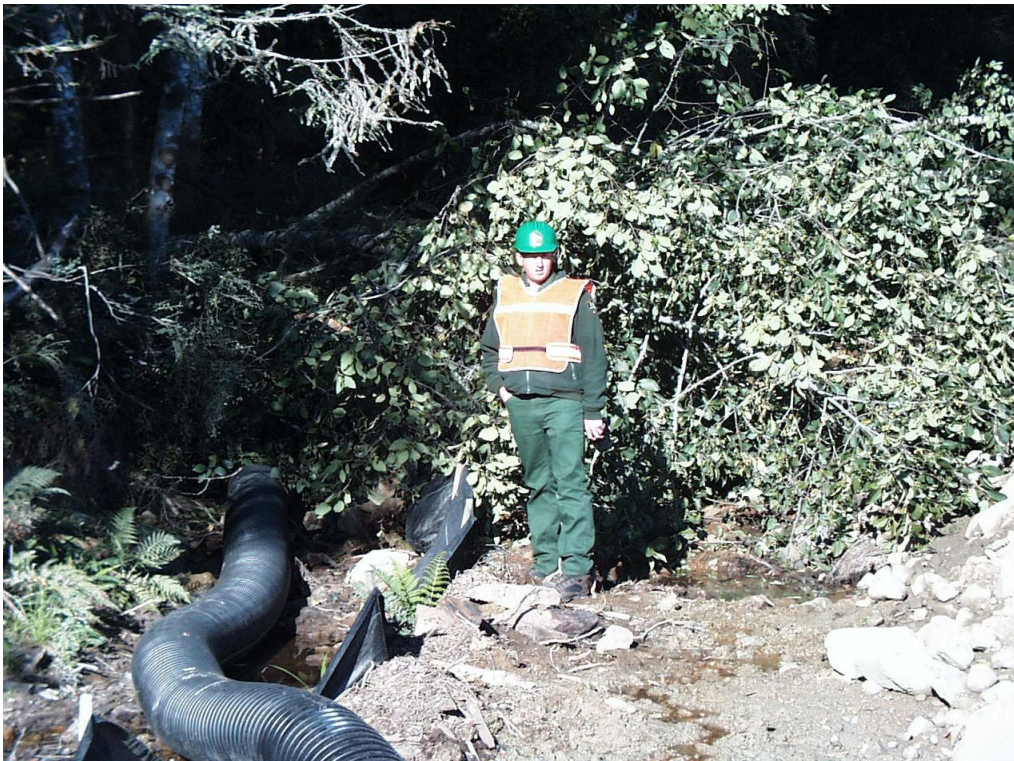
Photo 5. Inlet of diversion pipe with designer / builder (Dave Anderson, Fisheries Biologist).
