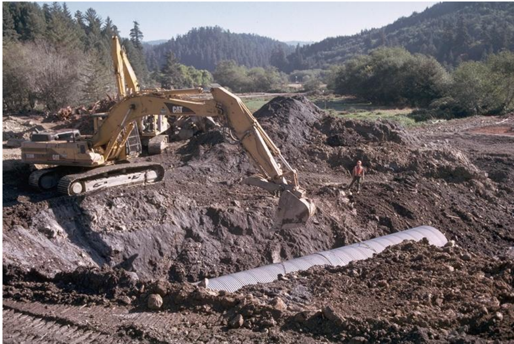
Photo 8. Installing new culvert for Davison Creek. Eight foot diameter culvert was buried half way, allowing channel bed to migrate vertically and horizontally.
