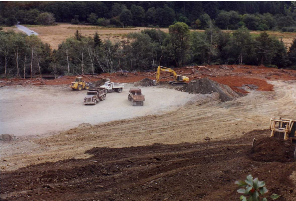
Photo 1. Trucks end hauling fill to parking lot site.
