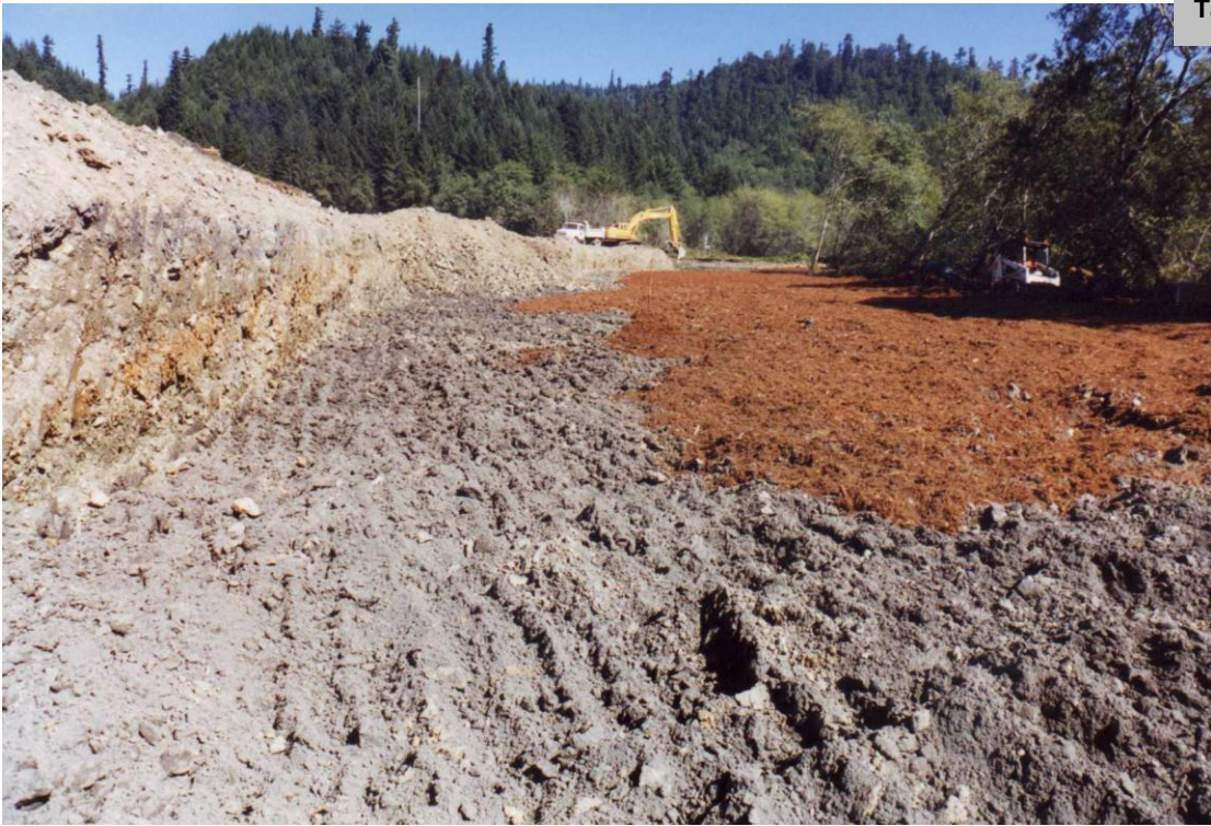
Photo 4. Original wetland soil surface contrasted with imported deck fill.
