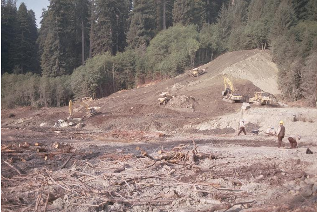
Photo 7. Large, Formidable Rocks (LFR's) at base of slope. Both excavators were required to move the boulders.
