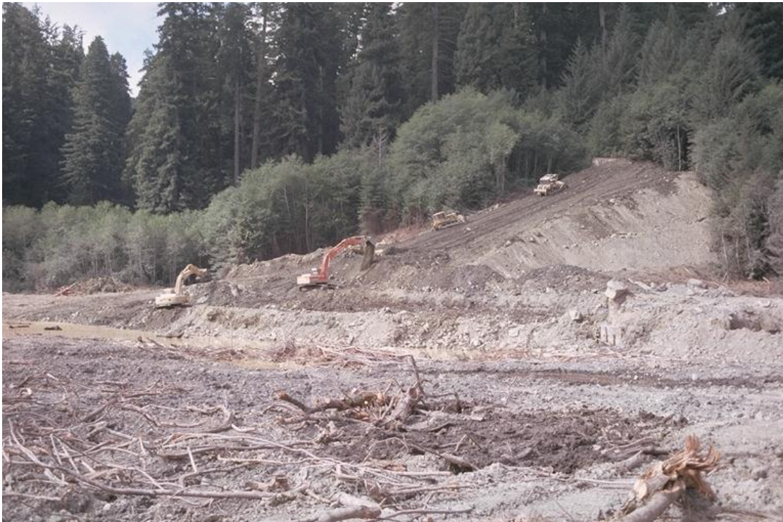
Photo 6. Multiple bailing effort to mix muck with dry fill. Note ponded water at base of excavation.
