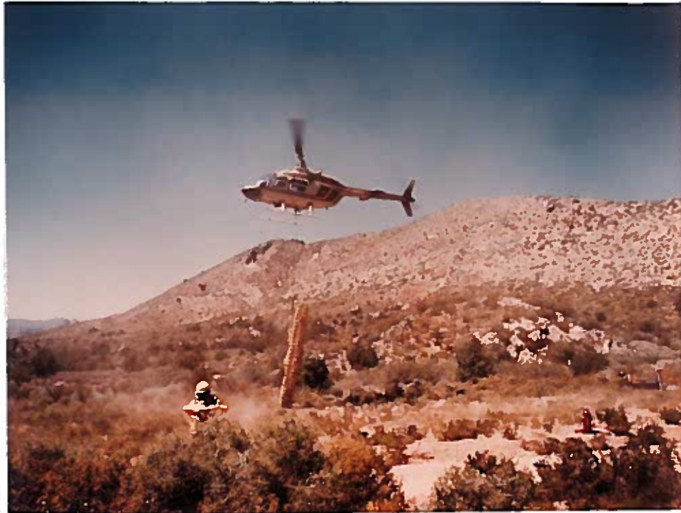
Figure 5. Helicopter slingloading construction materials to the Mirage Wildlife Catchment site, Virgin Mountains.
