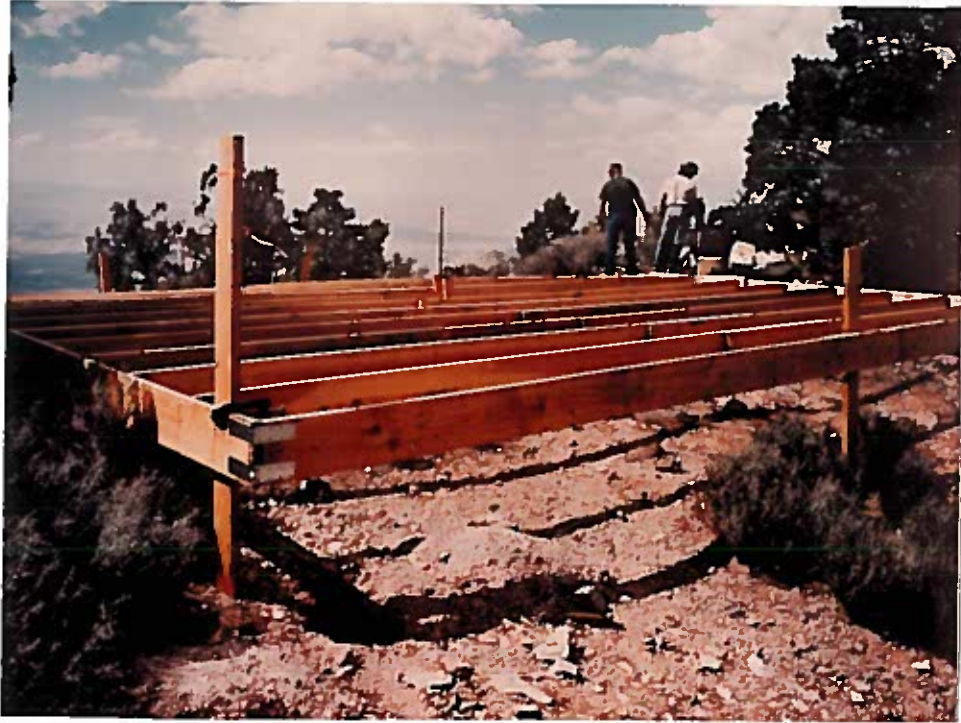
Figure 3. AGFD projects crew building the apron for Mirage Wildlife Water Catchments, Virgin Mountains.
