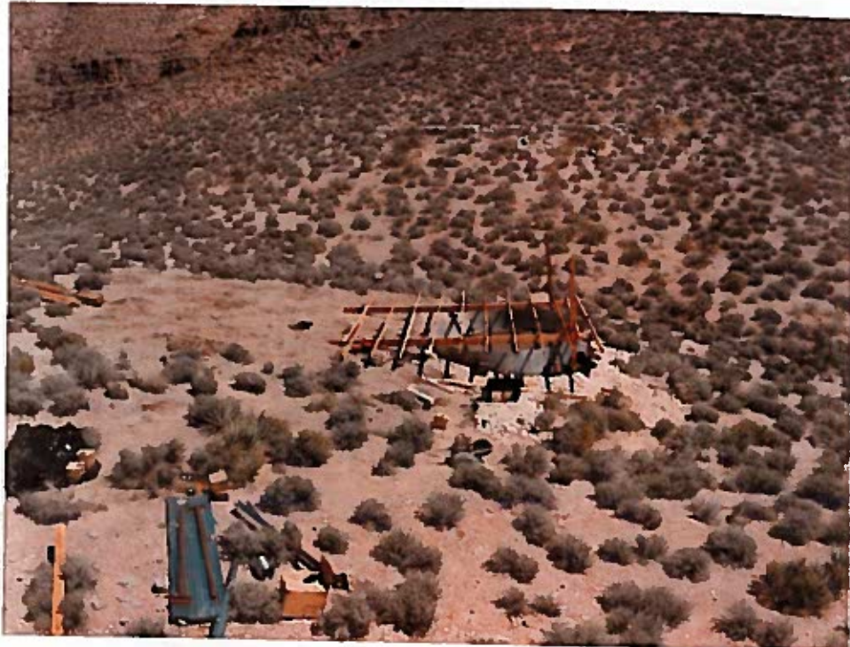
Figure 4. Overlook Wildlife Water Catchment during construction. Note placement of steel storage tank under apron, Grand Wash Cliffs.
