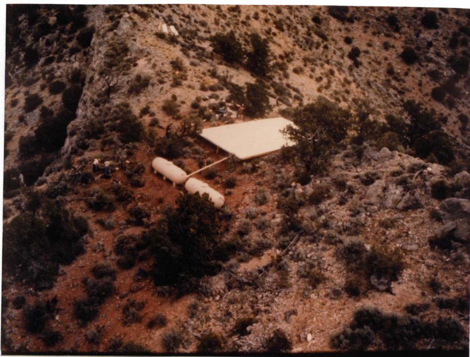
Mirage Catchment near completion prior to camouflage paint. Note topography and AGFD construction crew.
