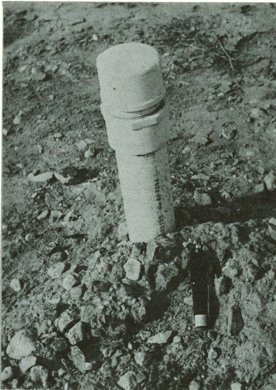
Figure 10. Close-up of upper end of soil moisture tube as installed on bank adjacent to channel at upper Ropes Draw Site showing plastic pipe with which hole is cased.
