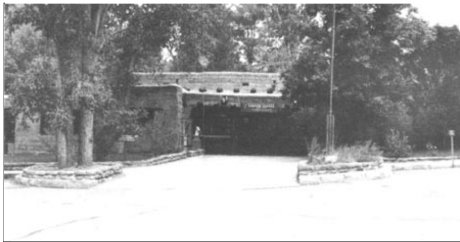
Figure 144. The front facade of the visitor center, 1988. Note the dense growth hiding much of the architecture.
