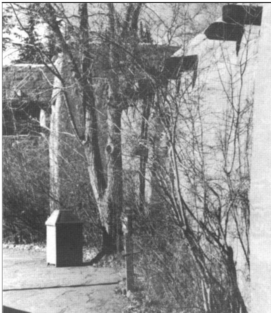
Figure 194. The parking area north wall, 1988. The box elder tree should be pruned up to raise the canopy.
