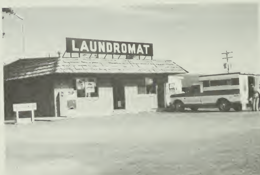
Photograph B Typical laundromat facilities at campground and motel developments.
