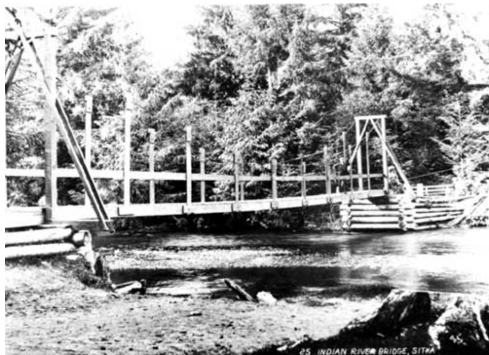
25 INDIAN RIVER BRIDGE, SITKA
