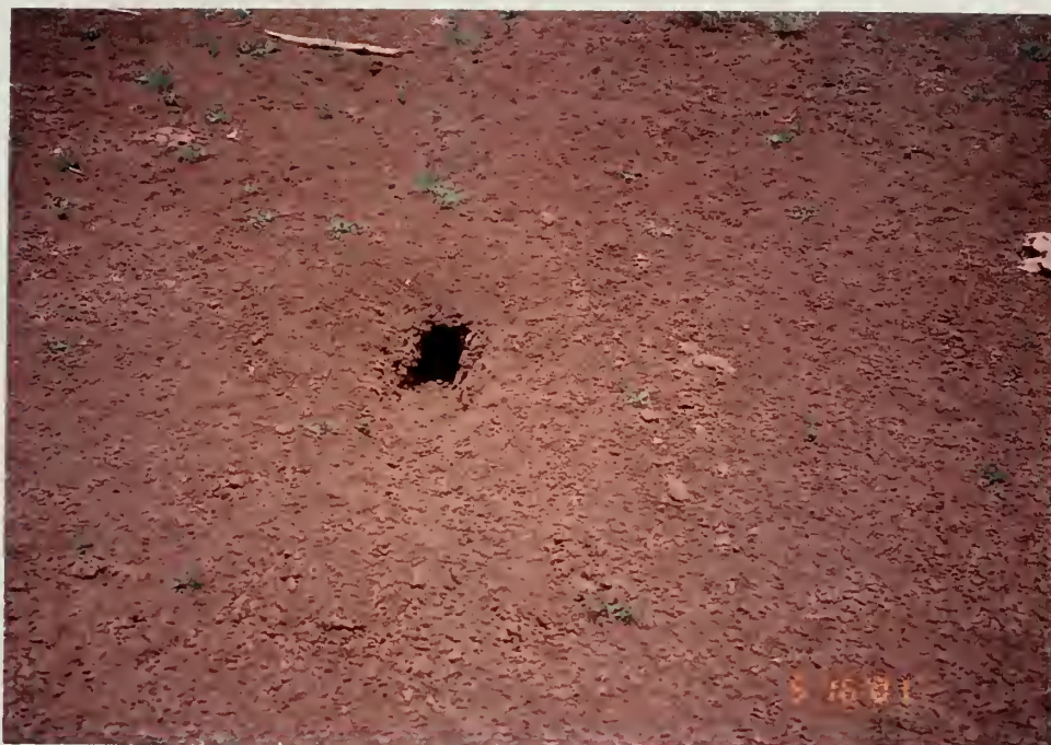
Photo 5. Hubbell Reservoir - Animal burrow on the upstream edge of the main embankment segment.
