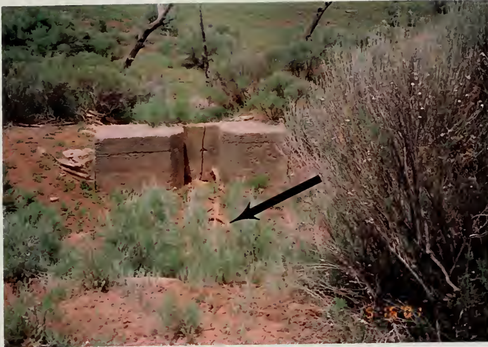
Photo 9. Hubbell Reservoir - Left reservoir inlet near the southwest corner of the reservoir, looking toward the reservoir. The arrow indicates the partially plugged inlet pipe. 5/16/01
