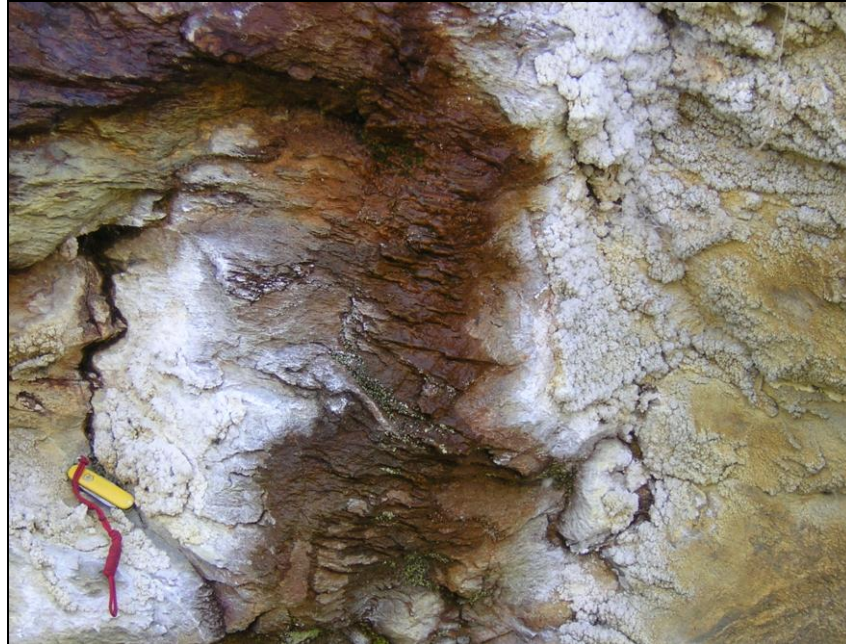
Figure B3. White gypsum blooms, and yellow (jarosite?) and dark orange oxide coatings on sulfidic metagraywacke exposed adjacent to the June 15, 1999 rockslide (CER-001) near Crabtree Meadows. The NNP test value for this rock was -22.02 as shown on Figure 1.
