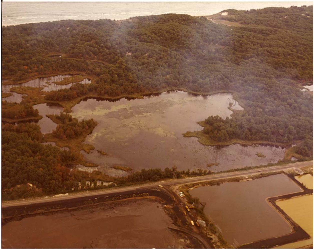
Photograph 2. Aerial photograph of the flooded Blag Slough with fly-ash settling ponds 11 and 12 in the foreground. Taken September 27, 1977.
