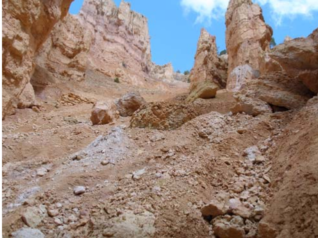
Figure 6a. Slope above Wall Street containing large amounts of loose debris.
