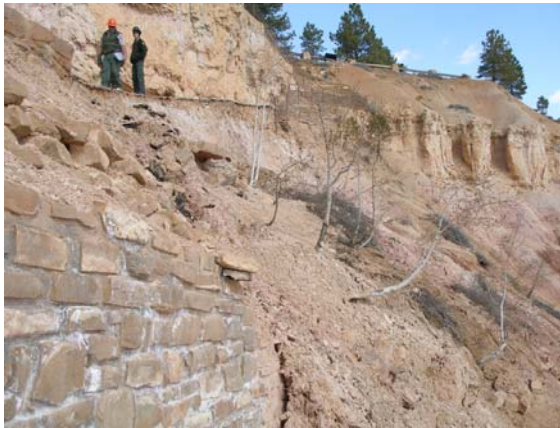
Figure 4a. The landslide with tension cracks, scarps and “pistol butted” aspen trees on the slope.
