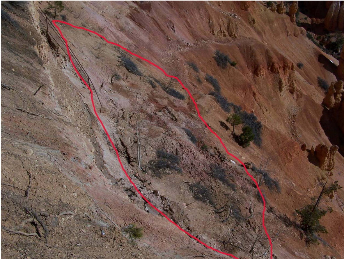
Figure 3. The landslide area below the asphalt section on the Navajo Loop Trail.
