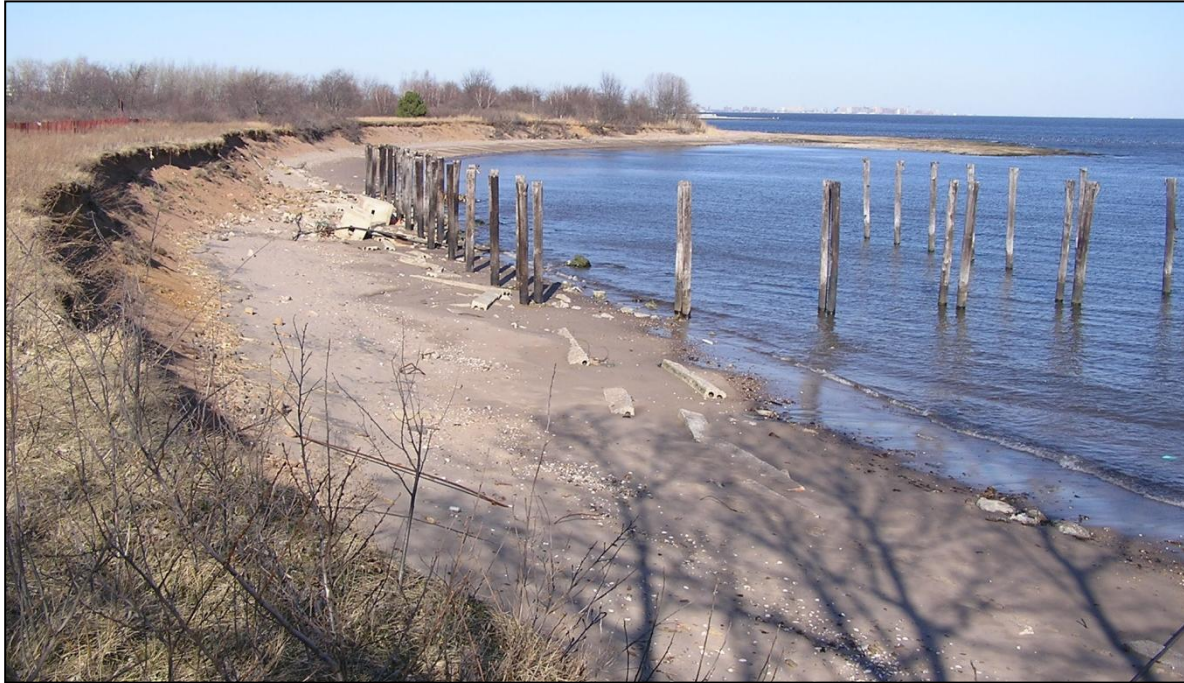
Figure 14. Severe erosion downdrift of projecting headland. Pilings are at site of demolished bath house. March 31, 2009.
