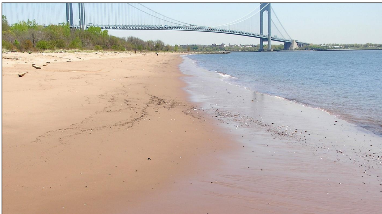
Figure 18. Beach-dune profile seaward of constructed sand dike, Fort Wadsworth. Glacial deposits are immediately inland of veneer of fill at this site. May 5, 2008.
