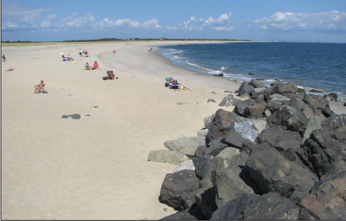
.Figure 11. Inland offset of shoreline downdrift of terminus of seawall, the Critical Zone, September 11, 2008.
