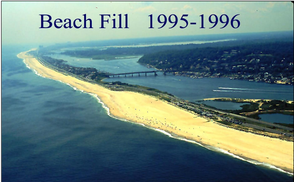
Figure 9. The artificially wide beach following beach nourishment at the Park entrance.
