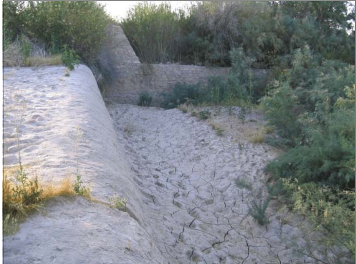
Dry plunge pool below the Wells-siding Diversion in July 2004.
