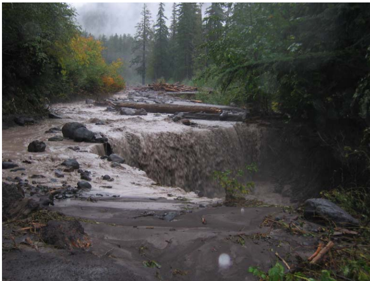
Figure 23. Fish Creek, following the September 29, 2005 debris flow flood, below debris flow deposit, just downstream where the creek crosses the West-side Road. See photo point in Figure 22.
