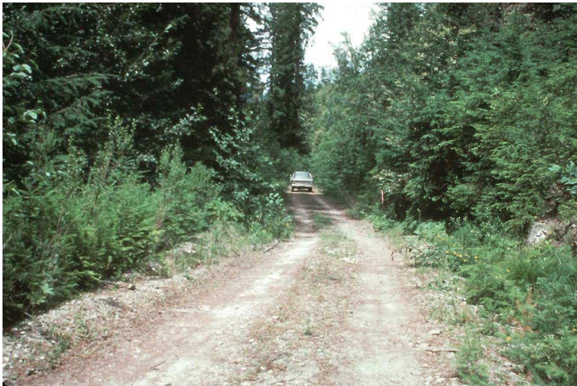
Unit: 86-5 Date: 7-2-1986, PP17, M-3-1-2 STA 88+00 pre HE outsloping, 35mm, (LEJ)
