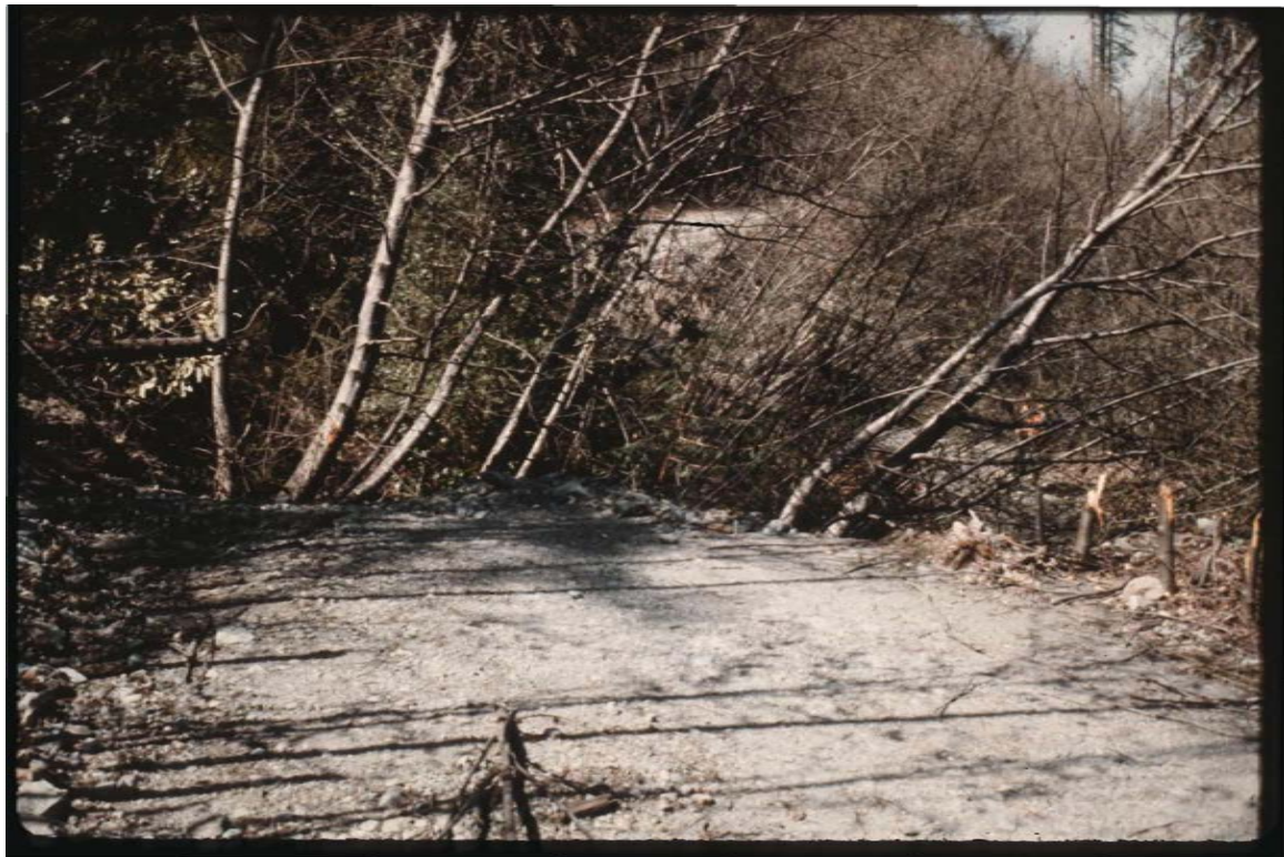
Unit: 83-2 PP#70 Landslide. 4/5/83
