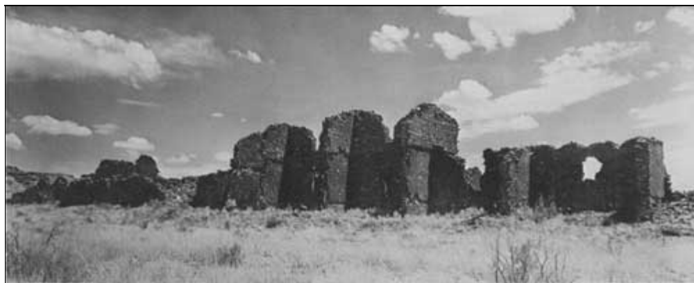
Kin Biniola—detached section. An impressive major ruin with interesting irrigation works and outstanding potential for interpretive use.
