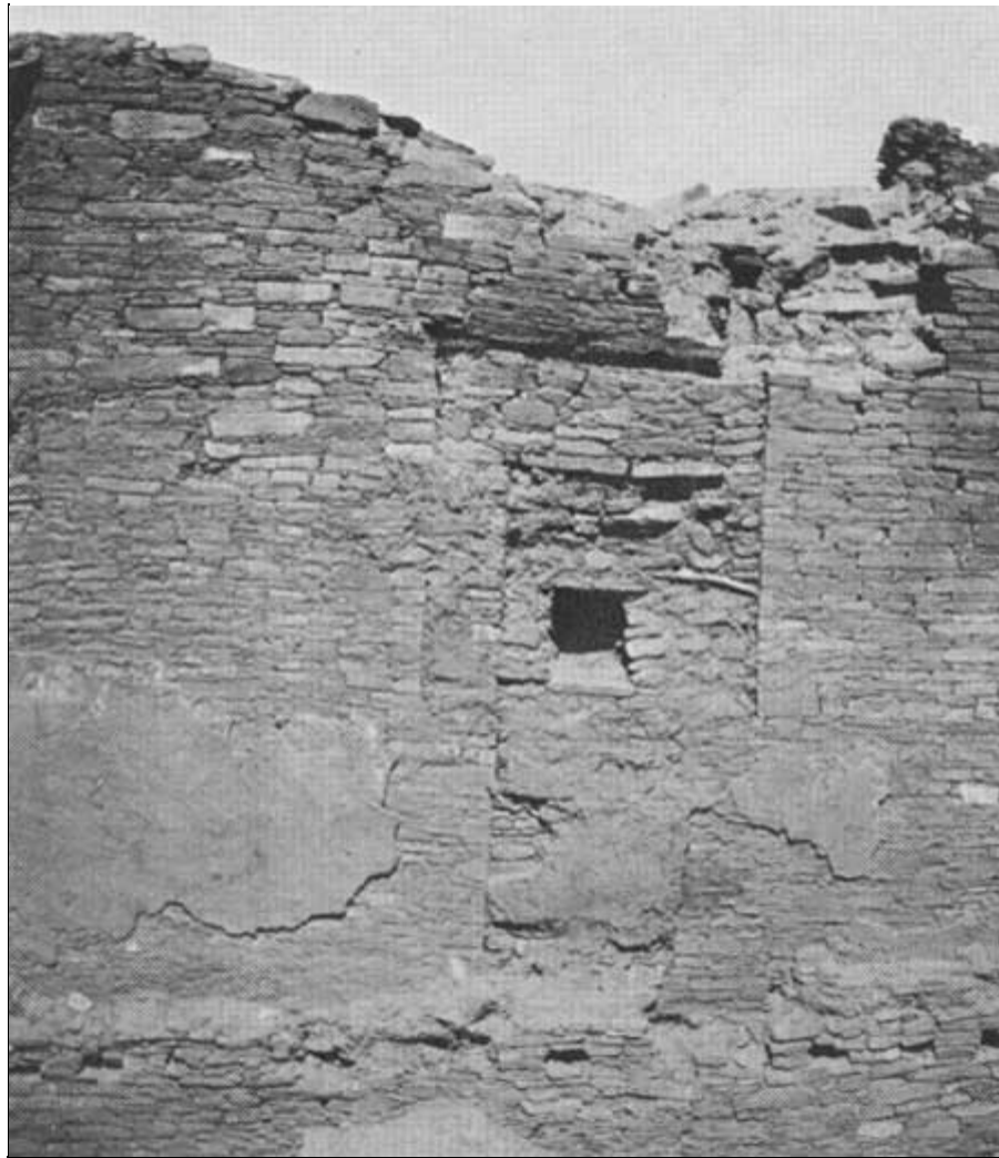
Ancient remodeling work. Original large T-doorway was partially closed and subsequently completely closed, but with a small storage alcove. Note prehistoric plaster and socket holes for floor beams of this second story room. ( Courtesy of the American Museum of Natural History )
