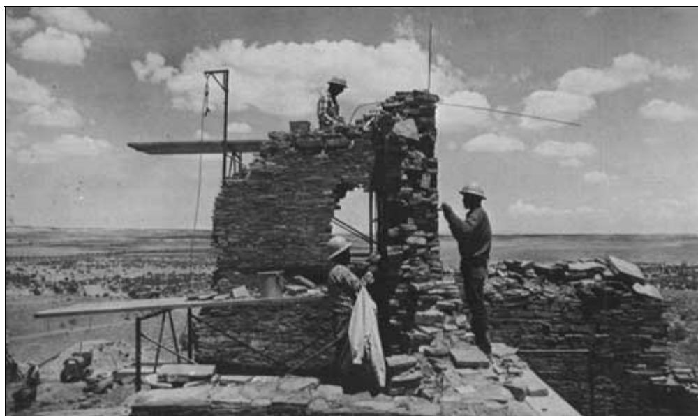
Ruins stabilization unit at work capping walls of Pueblo Pintado to prevent further deterioration.
