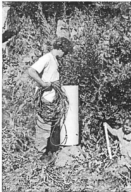
Figure 12. Installing stilling well to house a pressure transducer and thermistors to collect stream height and temperature data at the road culvert over Trauger's Creek.
