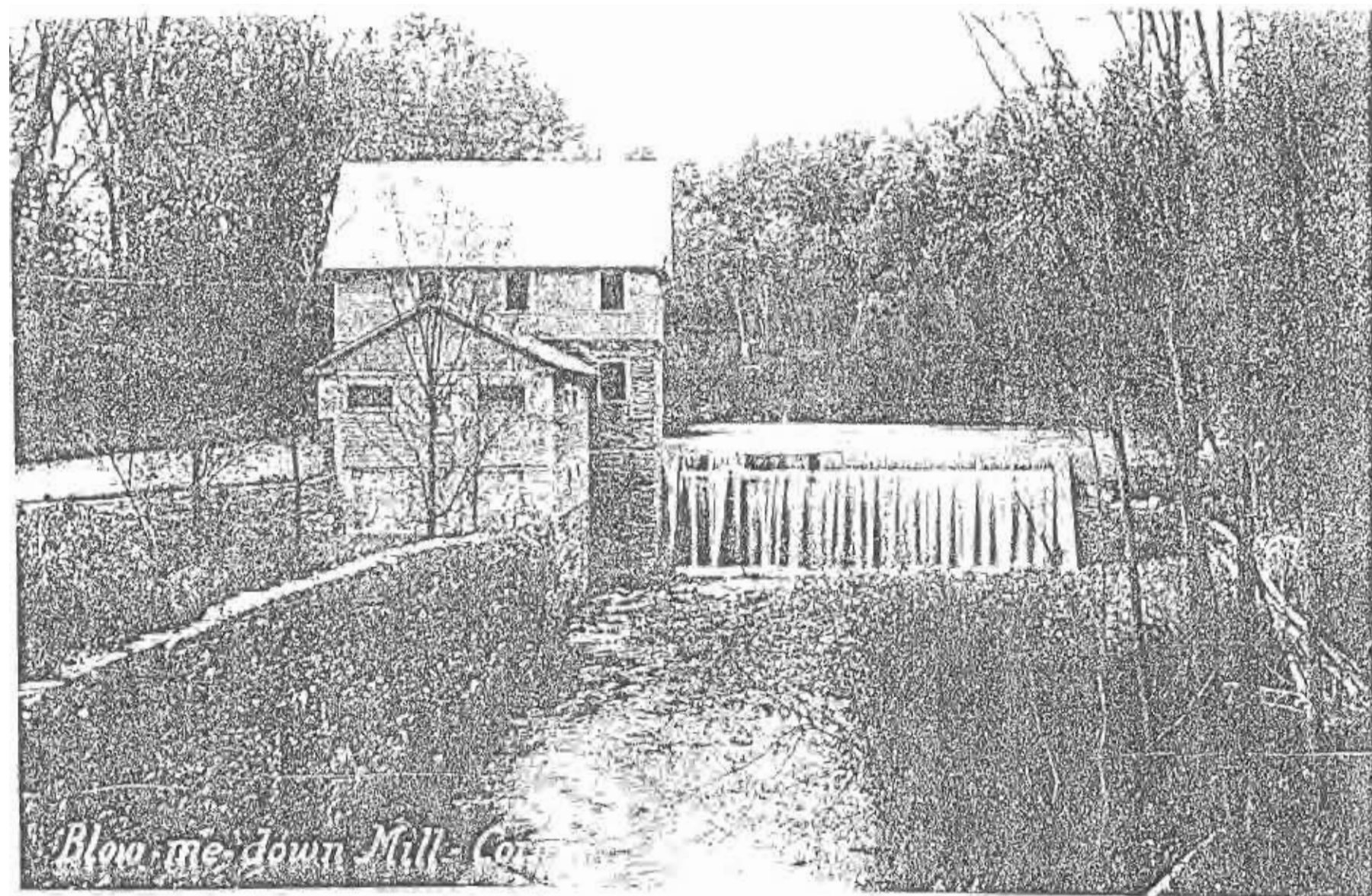
FIG. 23. Summer low-flow conditions at Blow-Me-Down Dam, around the turn of the century.
