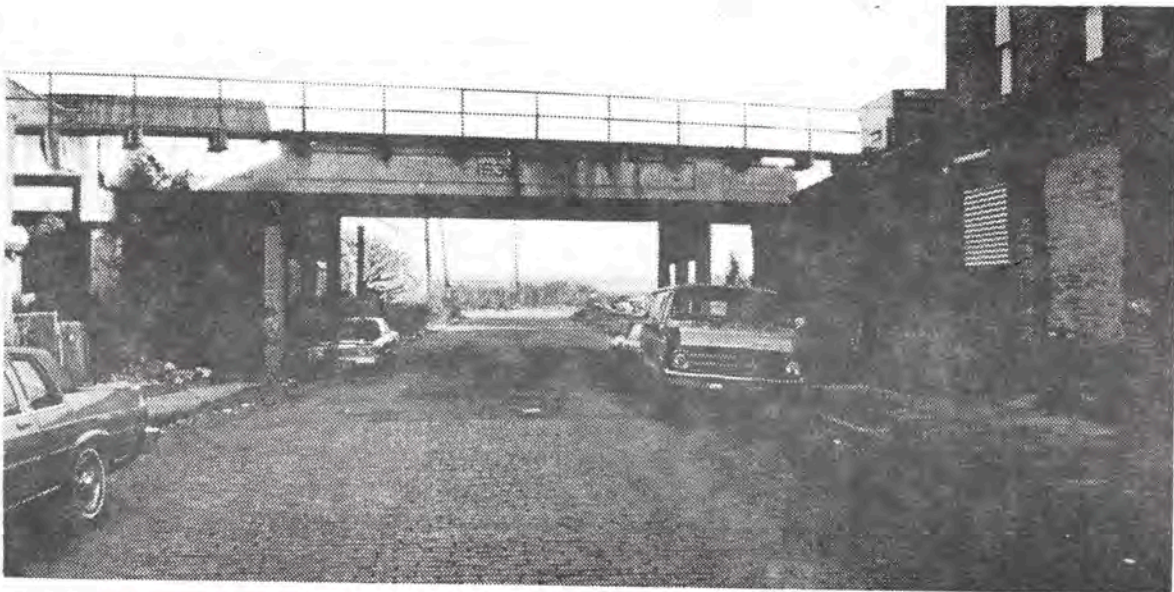
23. Raised SIRT tracks allowing vehicular access to the waterfront.
