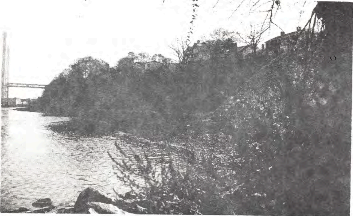
24. Steep Slopes limit pedestrian and vehicular access.
