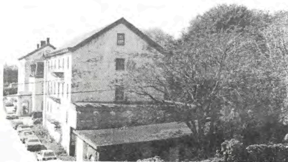
10, 11. View of Coast Guard site historic buildings from the water's edge and from access road along southern ferry terminal ramp.
