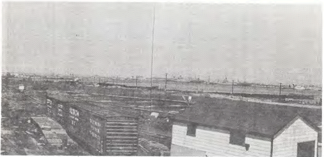
6,7 Chessie Railroad site. View from Richmond Terrace Esplanade, and below at vacant site.
