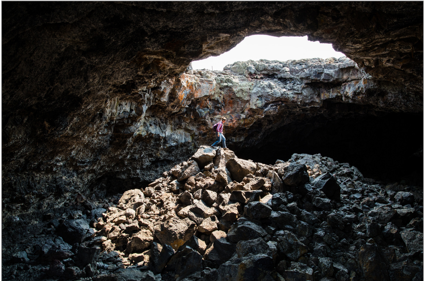
Collapse in Indian Tunnel, Craters of the Moon National Monument and Preserve. NPS / JACOB W. FRANK
