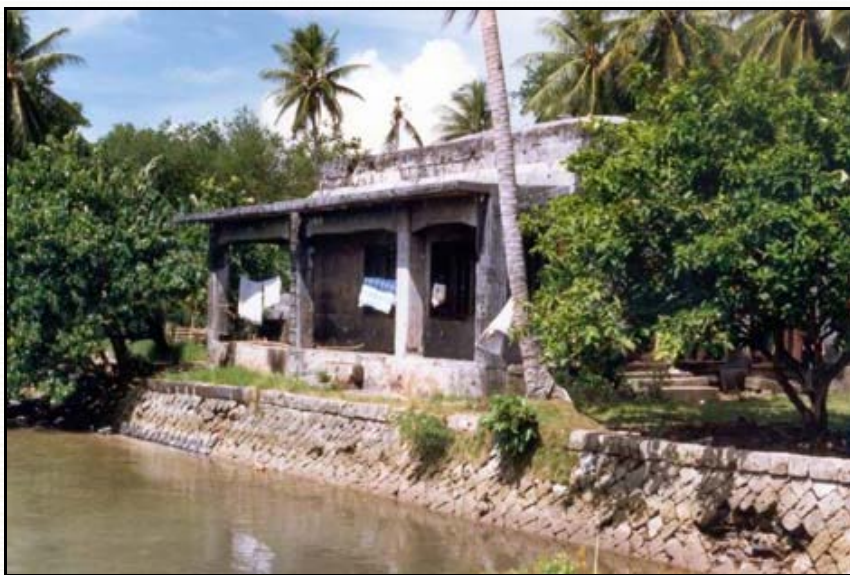
Figure 8. The old Japanese operations building on Dublon is now used as a residence. Note the precision Japanese Naval Base rockwork of the seawall.
