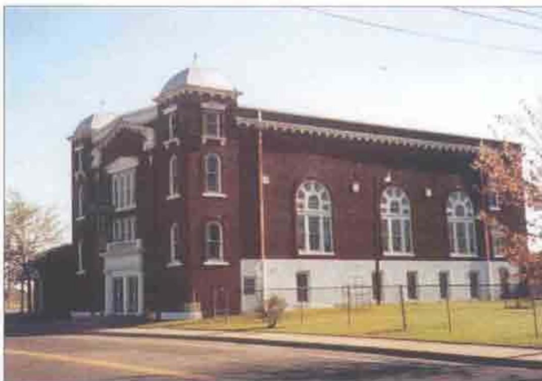
North and West (front) Facades.
