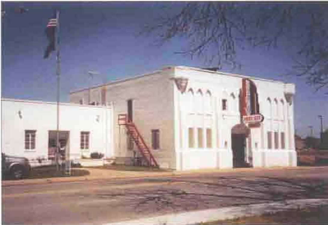
Front and west facades of the Tulsa National Guard Armory.
