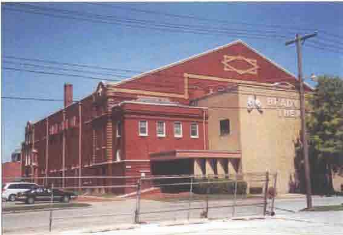
Front and southeast facades of the Tulsa Convention Center.
