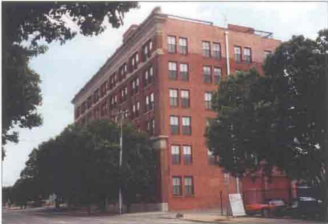
Front and west façade of Tulsa Tribune Building.
