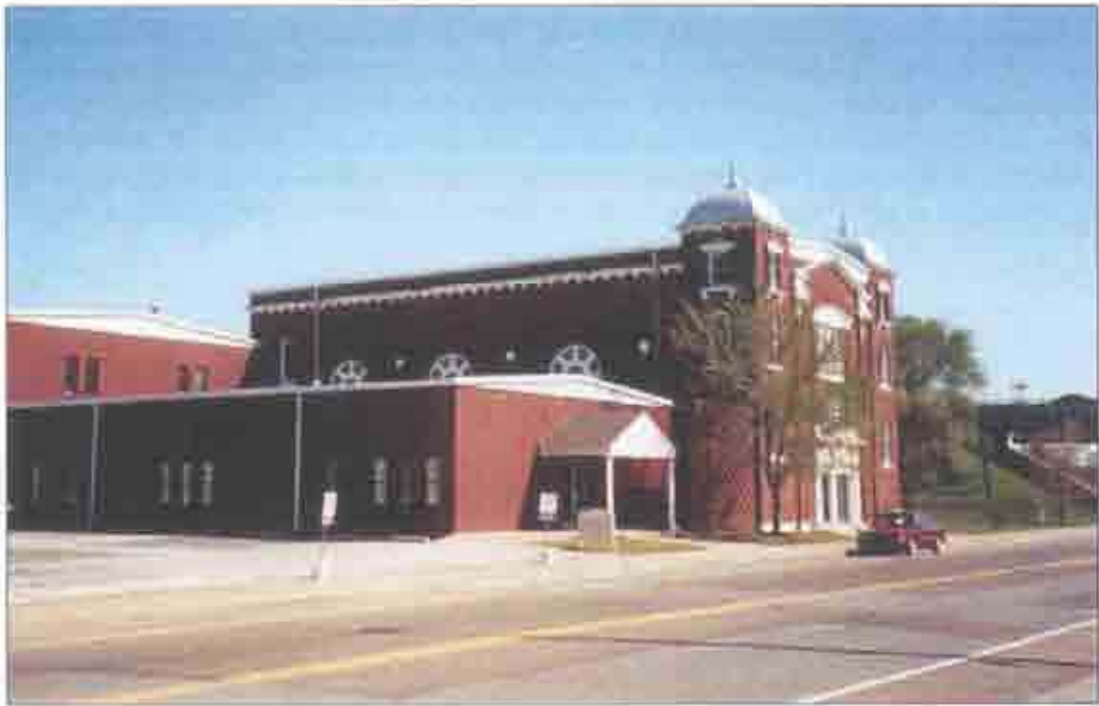
South and West (Front) Facades Showing 1970s-era Addition.
