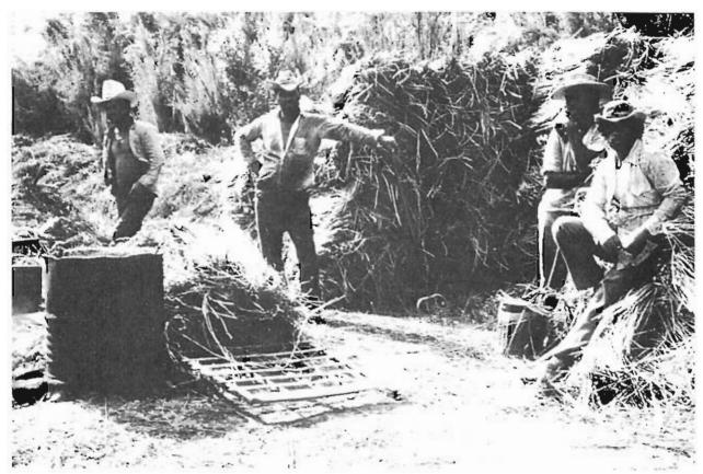
Fig. 41. Candelilleros watching a cameraman. The vat has received a heavy charge of weed, but the grates are still open. Lower Canyons.
