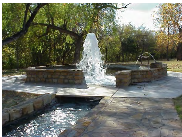
Figure 11. Vendome Well and Flower Park in Chickasaw National Recreation Area. When drilled in 1922, Vendome Well became the largest artesian well in Oklahoma, producing 9,500 liters (2,500 gallons) of water per minute. The water is 99% fresh and 1% brine. Note the drinking fountain that allows visitors to drink from the well. National Park Service photograph, available at http://www.nps.gov/chic/learn/photosmultimedia/photogallery.htm (accessed 15 June 2015).
