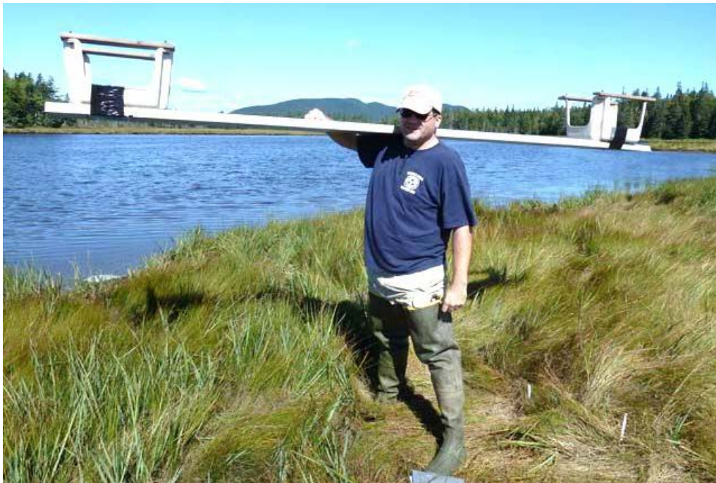
Figure 2.16. Temporary platform (Acadia National Park, ME, USA).
