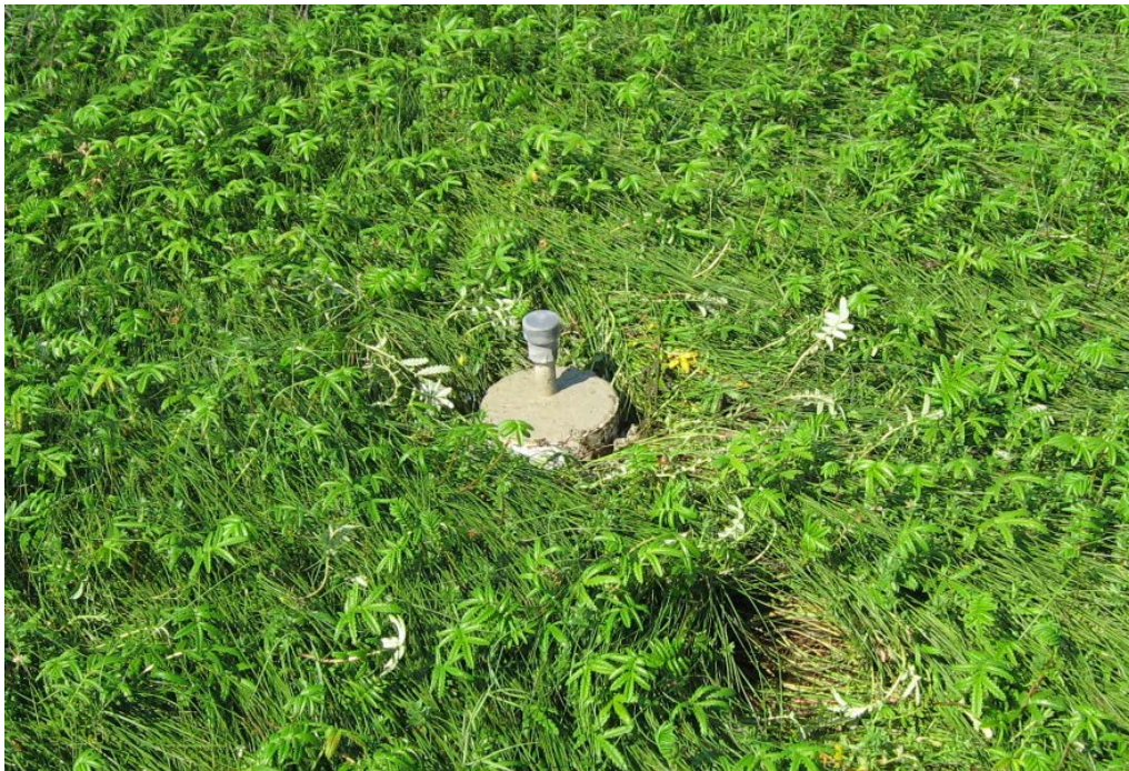
Figure 3.28. Completed deep SET mark.
