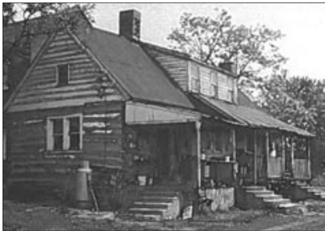
Like most early Montgomery County residences, Chiswell is constructed of chestnut logs. (Chiswell Place, Damascus, MD)
