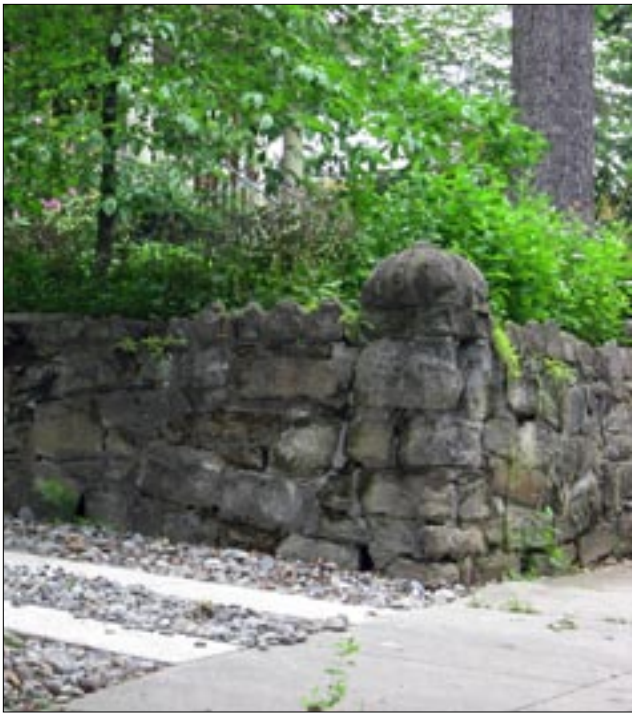
Guideline 13.1: Replace only those portions of a retaining wall that are deteriorated.
