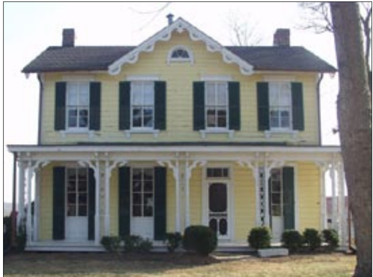
This Gothic Revival house is highly decorative with elaborate porch columns and brackets. (Gassaway, Germantown vicinity)
