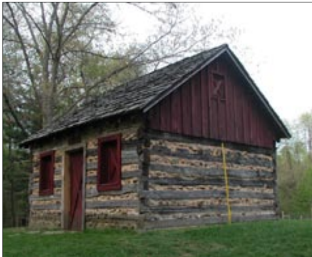
The majority of Montgomery County houses built in the mid- to late 18th century were constructed of logs. (Locust Hill, Brookville, MD)
