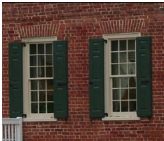
A gauged flat arch lintel is a characteristic of the Georgian style. (Locust Grove, Bethesda vicinity)
