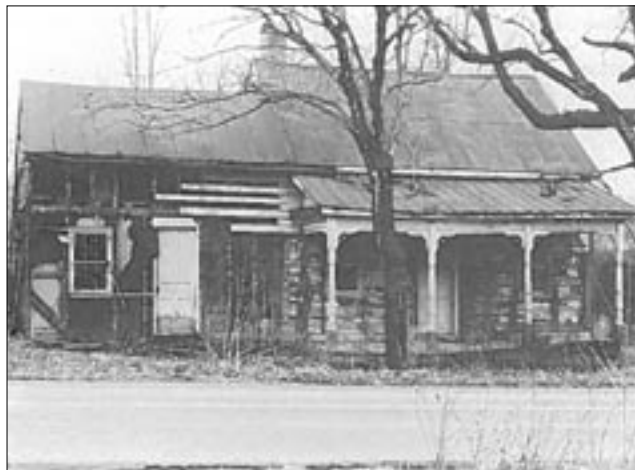
This house displays the use of braced framing, a common building technique in the early 19th century. (Hyattstown, MD)
