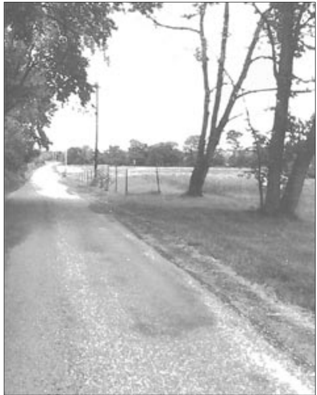
Martinsburg Road is a surviving one-lane paved road. The road was paved in 1931. (Poolesville, MD)
