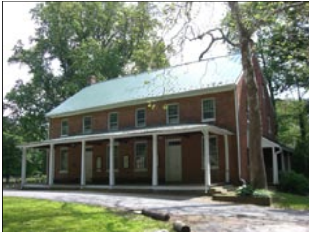
Federal style houses have low pitched roofs and symmetrical facades. (Sandy Spring Friends Meeting)
