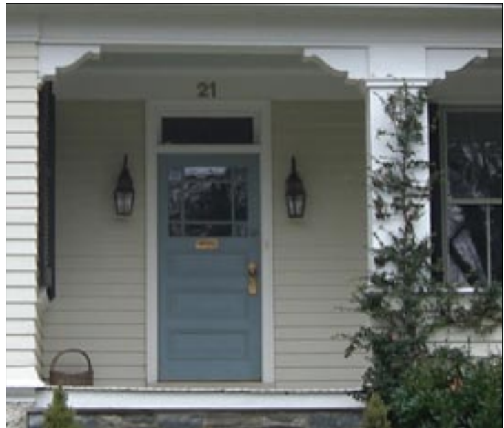
Craftsman style houses are commonly clad with wood clapboard.
