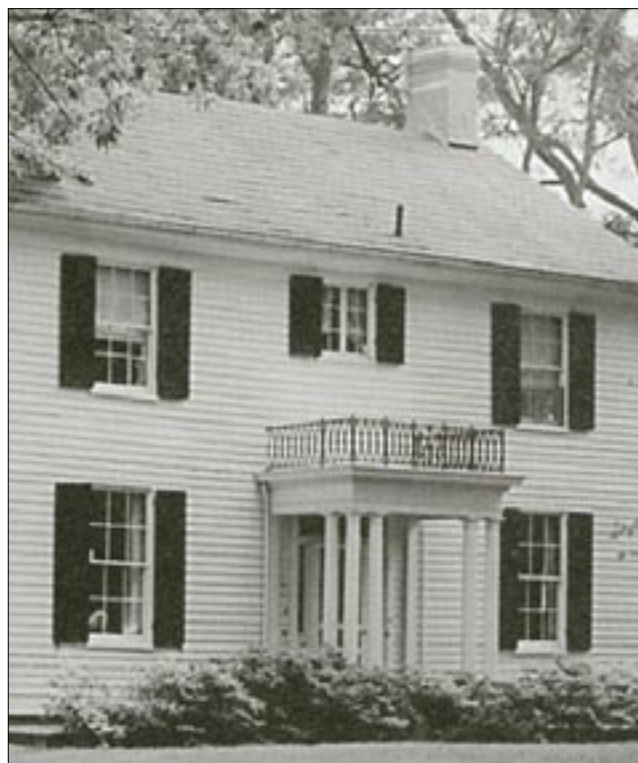
Windows in the Greek Revival style are typically six-over-six. (Samuel Perry House, Bethesda)
