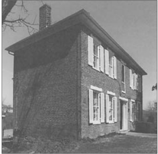
Historically, brick and masonry construction comprised a small percentage of the housing stock. (Mount Ephraim)
