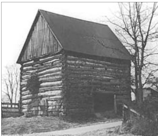
One of the last standing tobacco houses in Montgomery County. Located on the Brandenburg Farm, the structure was built in the mid-1800s. (Damascus, MD)
