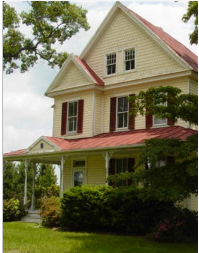
A turret is a common characteristic of the Queen Anne style, as is the ornate wood work. (Jacob Allnut House, Laytonsville vicinity)
