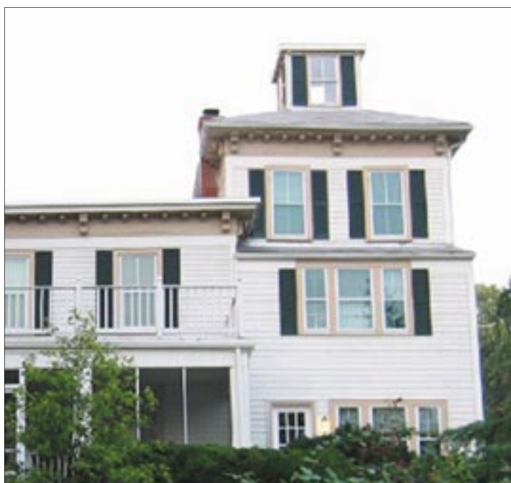
Ornate treatment of the eaves, including the use of brackets and dentil courses are characteristics of the Italianate style. (Lawrence House, Linden, MD)
