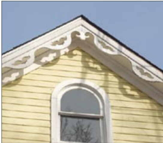
Elaborate finishes are typical of the Gothic Revival style. This house has a "gingerbread" vergeboard. (Gassaway, Germantown vicinity)
