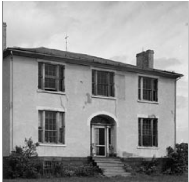
A front entrance with an elliptical fan light and flanking side lights are characteristics of the Federal style. (Montevideo, Potomac vicinity)
