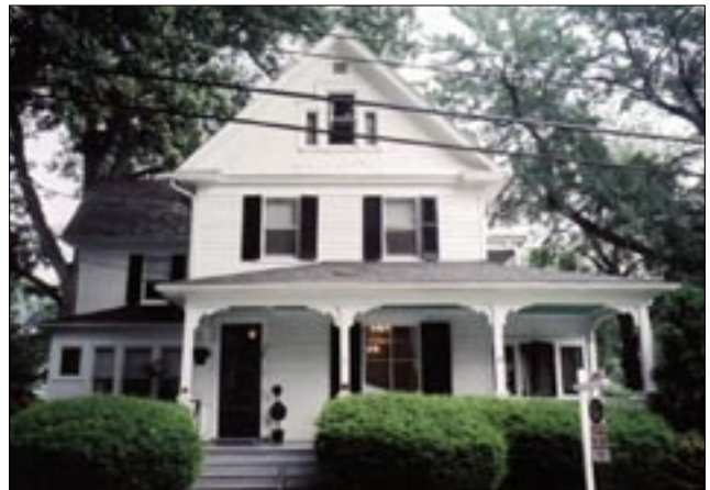
A full width porch is a common feature of the Victorian Vernacular style. (Cherry Chase Section Five)
