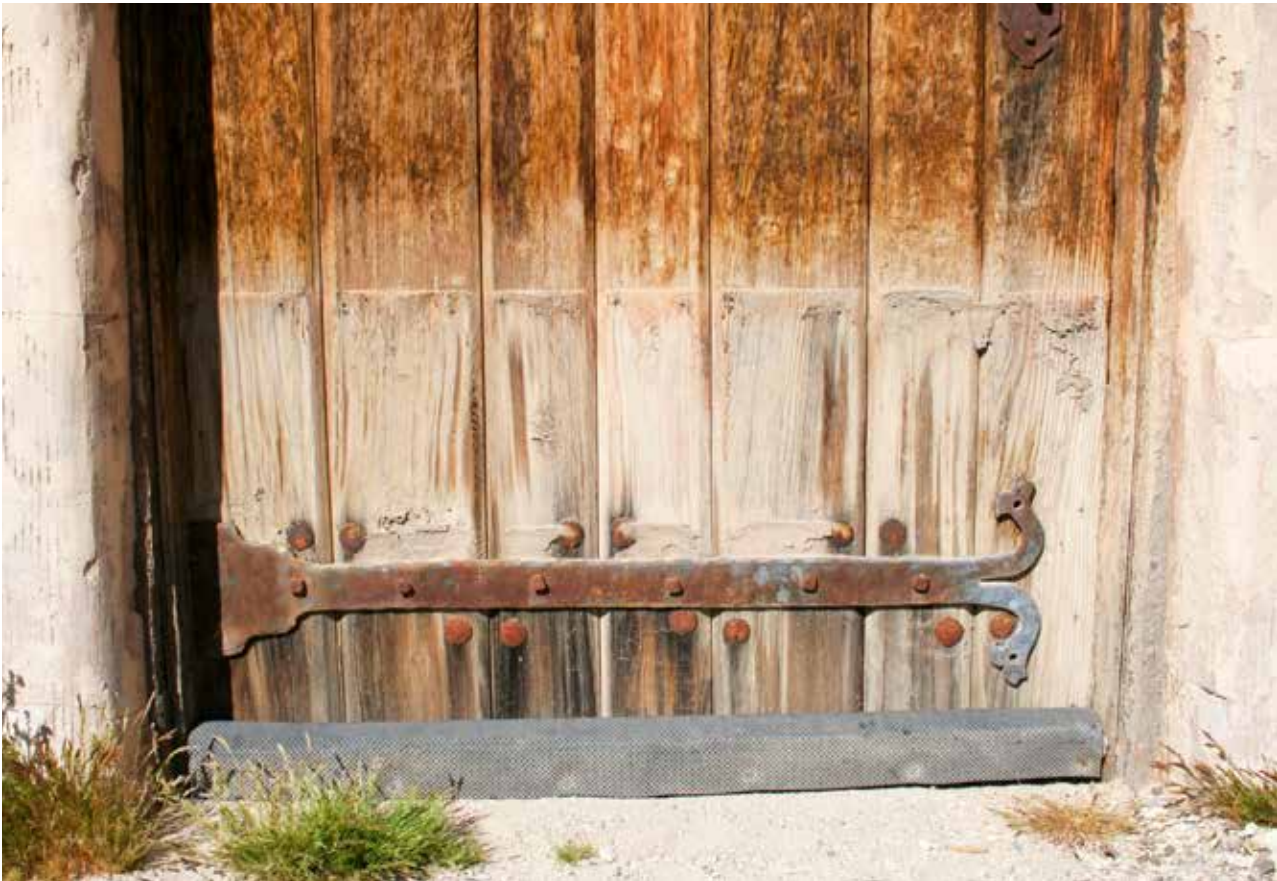
Figure DEVA 1.8: Evidence of moisture staining and sediment deposits on the south stable door and hardware, detail view, seen as a flood impact in the Scotty's Castle building complex. (Kerr/UO CLRG, 2016)
