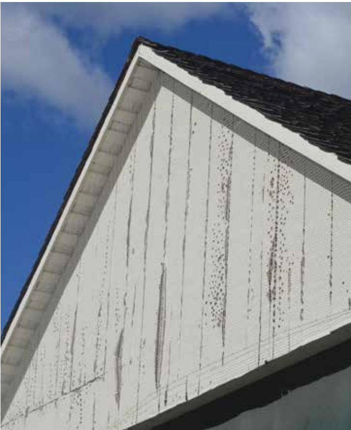
Figure EUON 1.8: Woodpecker bore-holes are evident across the west gable of the Old Barn. Note synthetic mesh netting, hung to deter further damage. (Malinay/UO CLRG, 2016)
