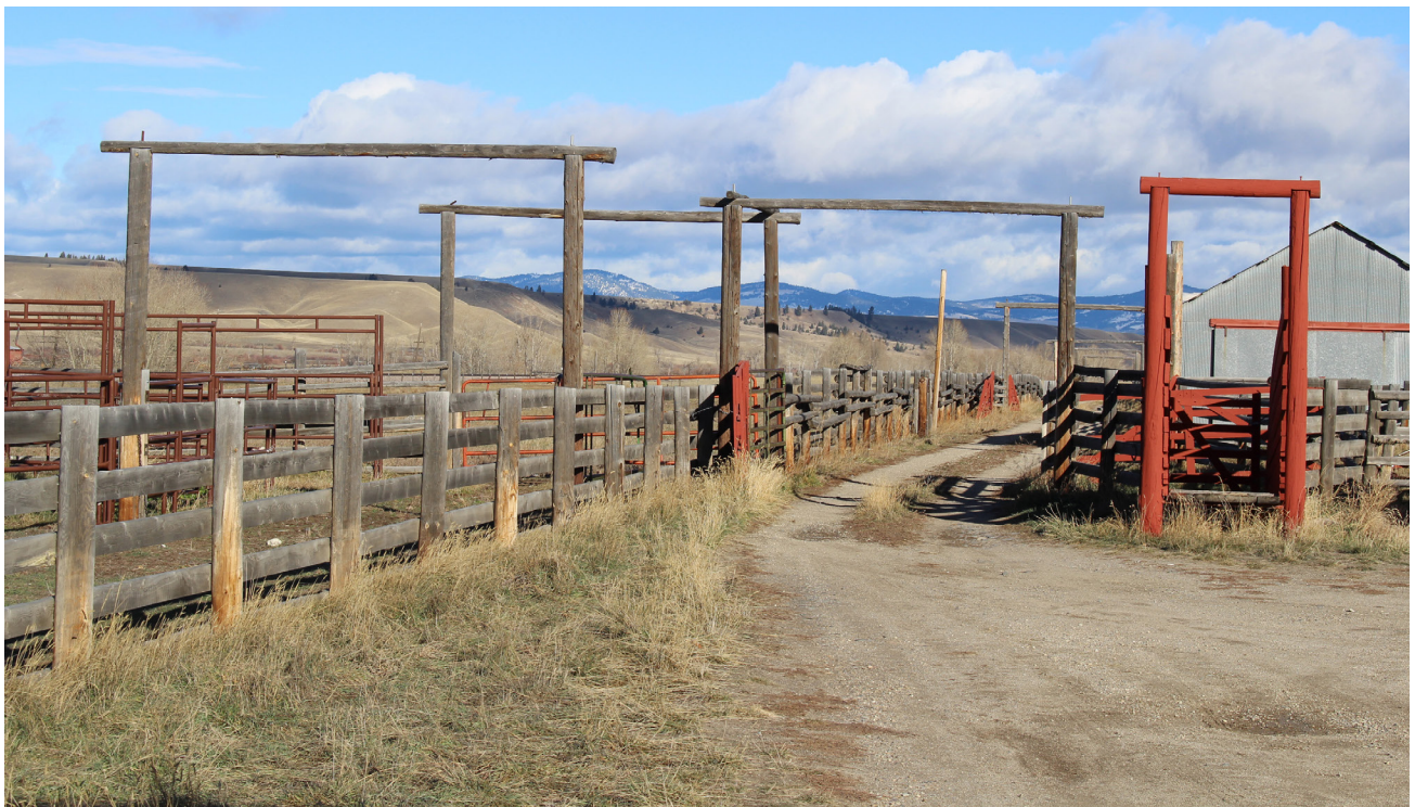
Figure 1-6. The East Feed Lot / Warren Hereford Ranch component landscape is an organized grid of feedlots, sheds, and barns, situated on the level, elevated plain east of the Clark Fork River. (Mundus Bishop, 2015)
