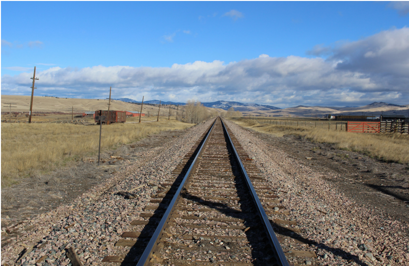
Figure 1-10. The Railroad Corridor and Barrow Pit/Wetland component landscape includes the double set of railroad tracks that traverse the ranch north - south, and the barrow pits that were created as part of the railroad grade construction. (Mundus Bishop, 2015)
