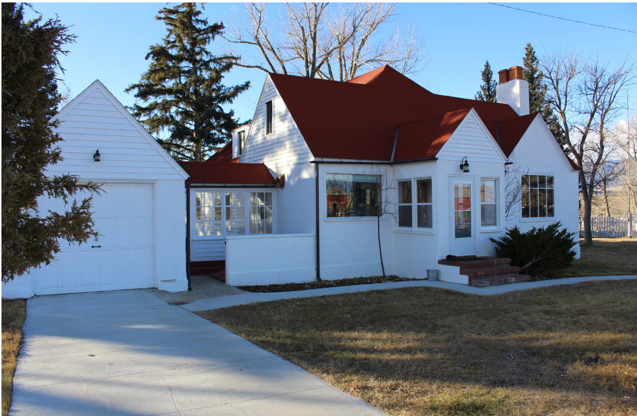
Figure 1-8. The Warren Residence component landscape includes the Warren Residence, outbuildings, vegetation, and small scale features constructed by Conrad Warren. (Mundus Bishop, 2015)
